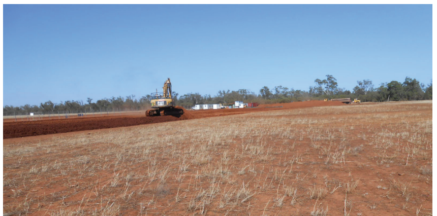
Construction underway at the Nyngan site
