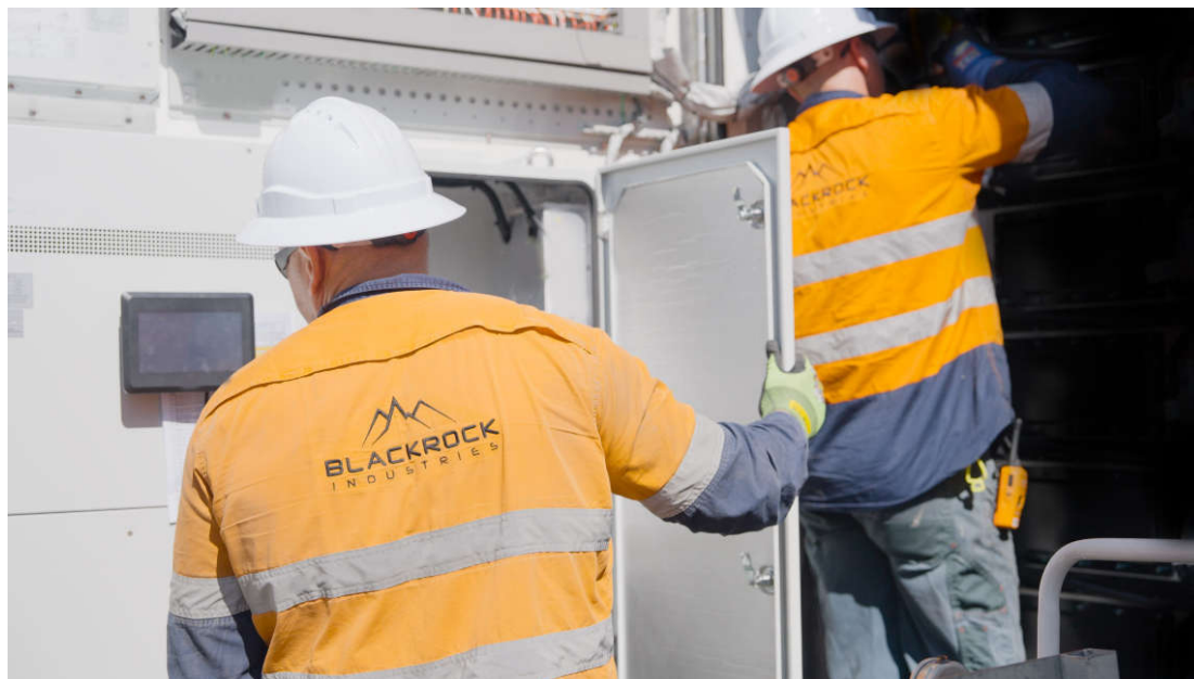
Blackrock contractors working on a battery cell at Liddell Battery, NSW
