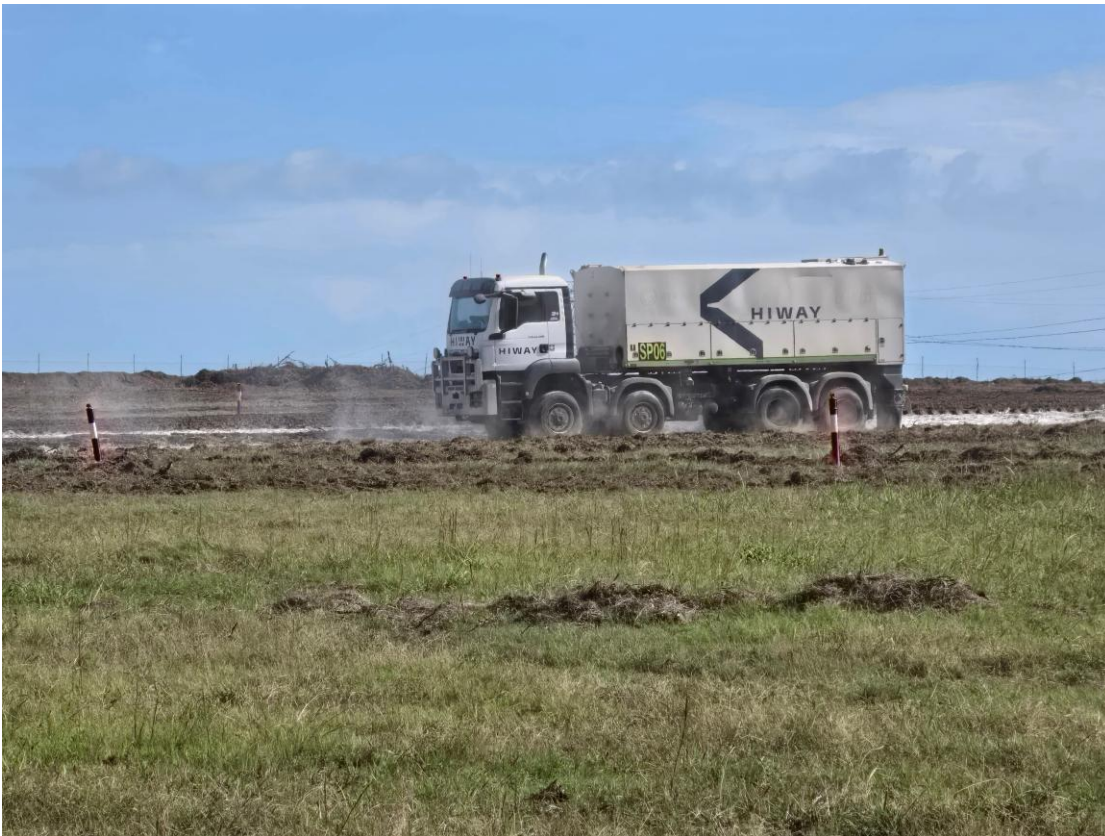
Plate 24 – Acid Sulfate Soil being treated
