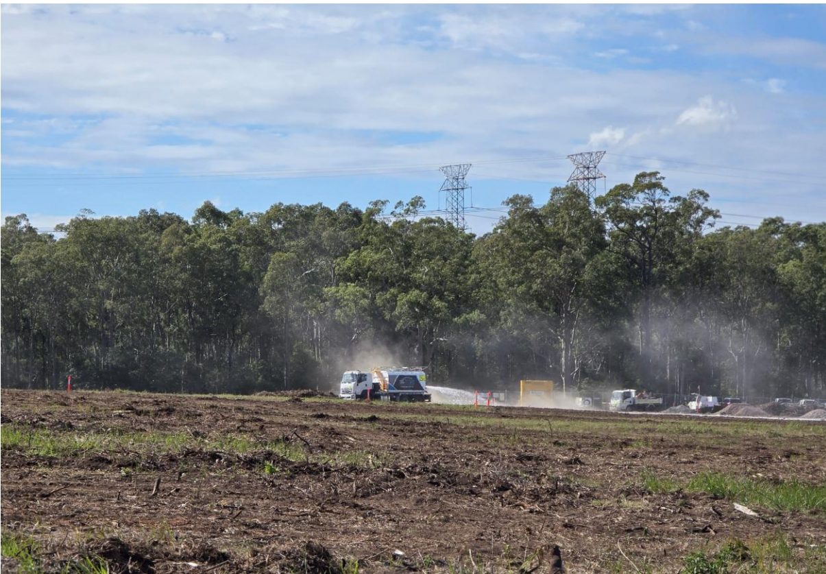
Plate 18 – Watercart in operation for active Acid Sulfate Soil treatment area
