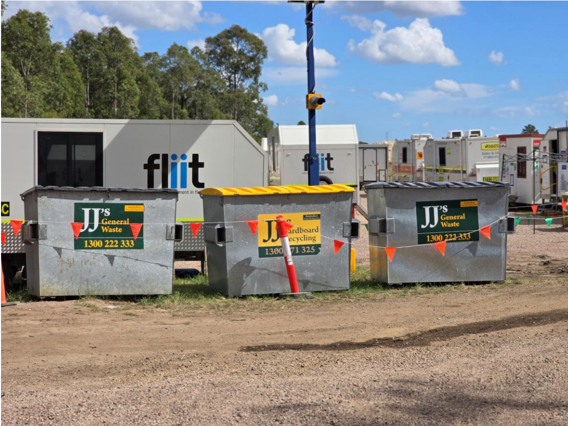
Plate 34 – Segregated bulk waste bins at temporary site offices area
