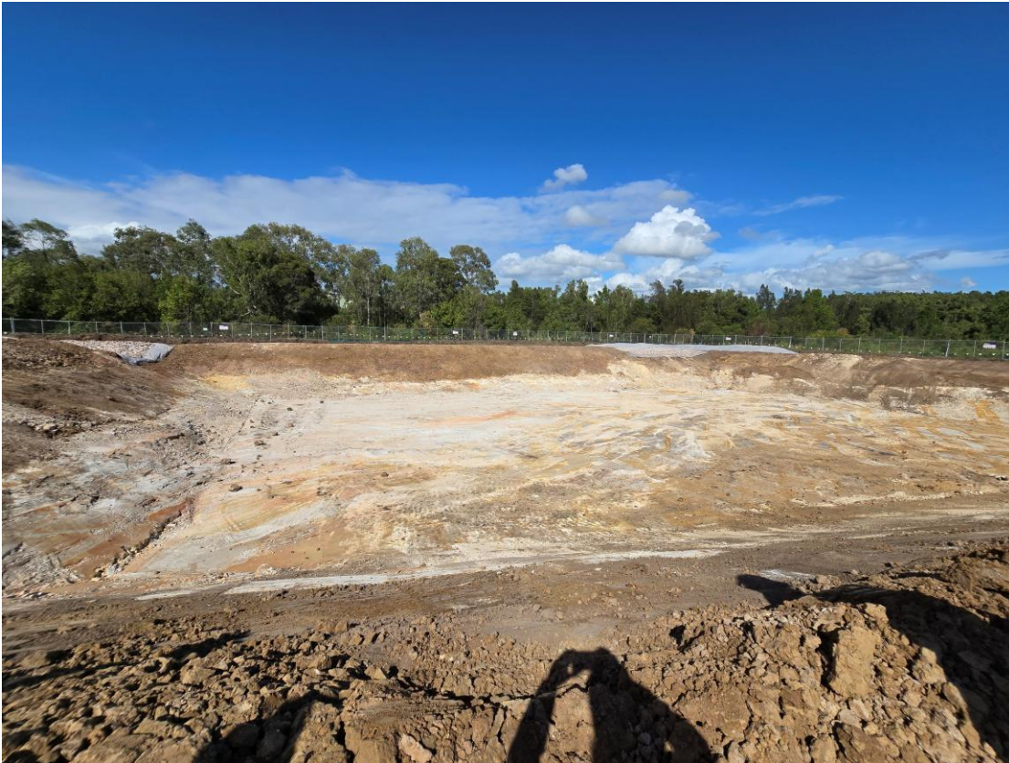
Plate 21 – Southern Water Basin being constructed
