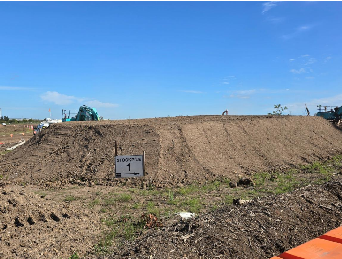
Plate 16 – Treated topsoil stockpile with signage in place
