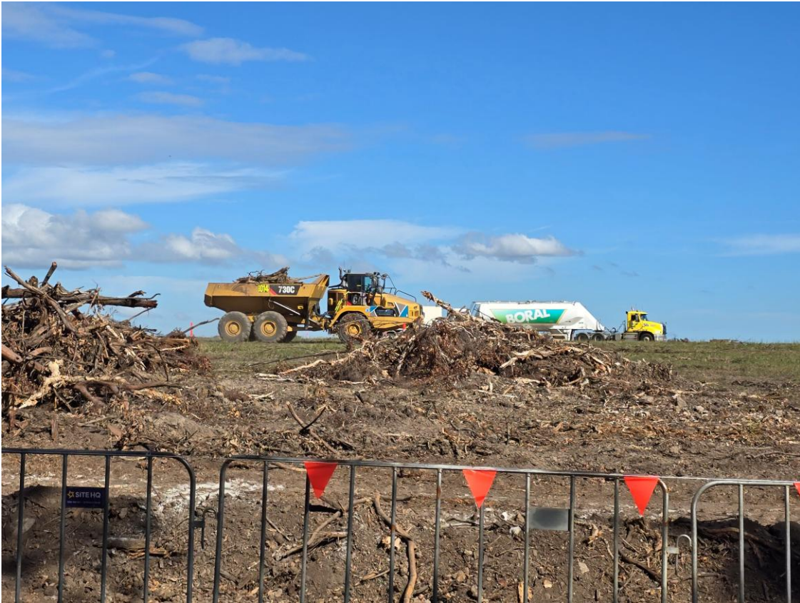
Plate 1 - Equipment operating within the clearing and grubbing work area
