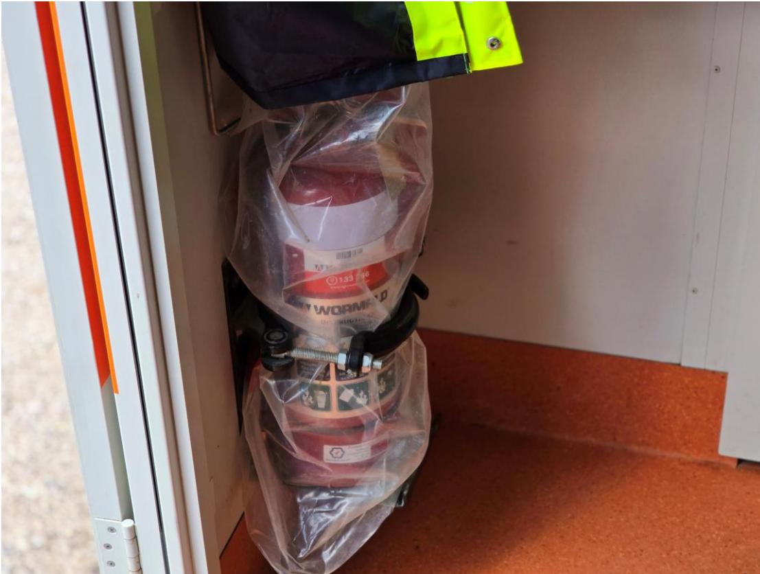
Plate 33 – Portable fire extinguisher in office
