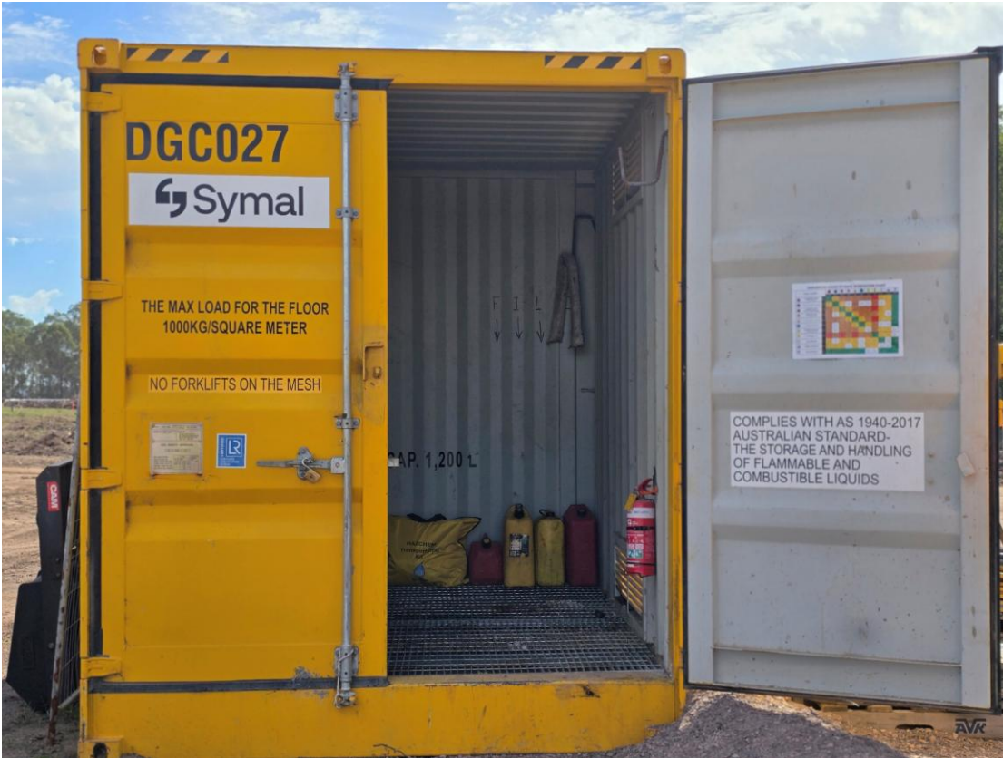
Plate 25 – Dangerous goods storage container
