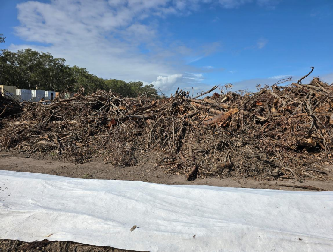
Plate 15 – Stockpiled vegetation to be used for mulch and placement along the Project disturbance boundary
