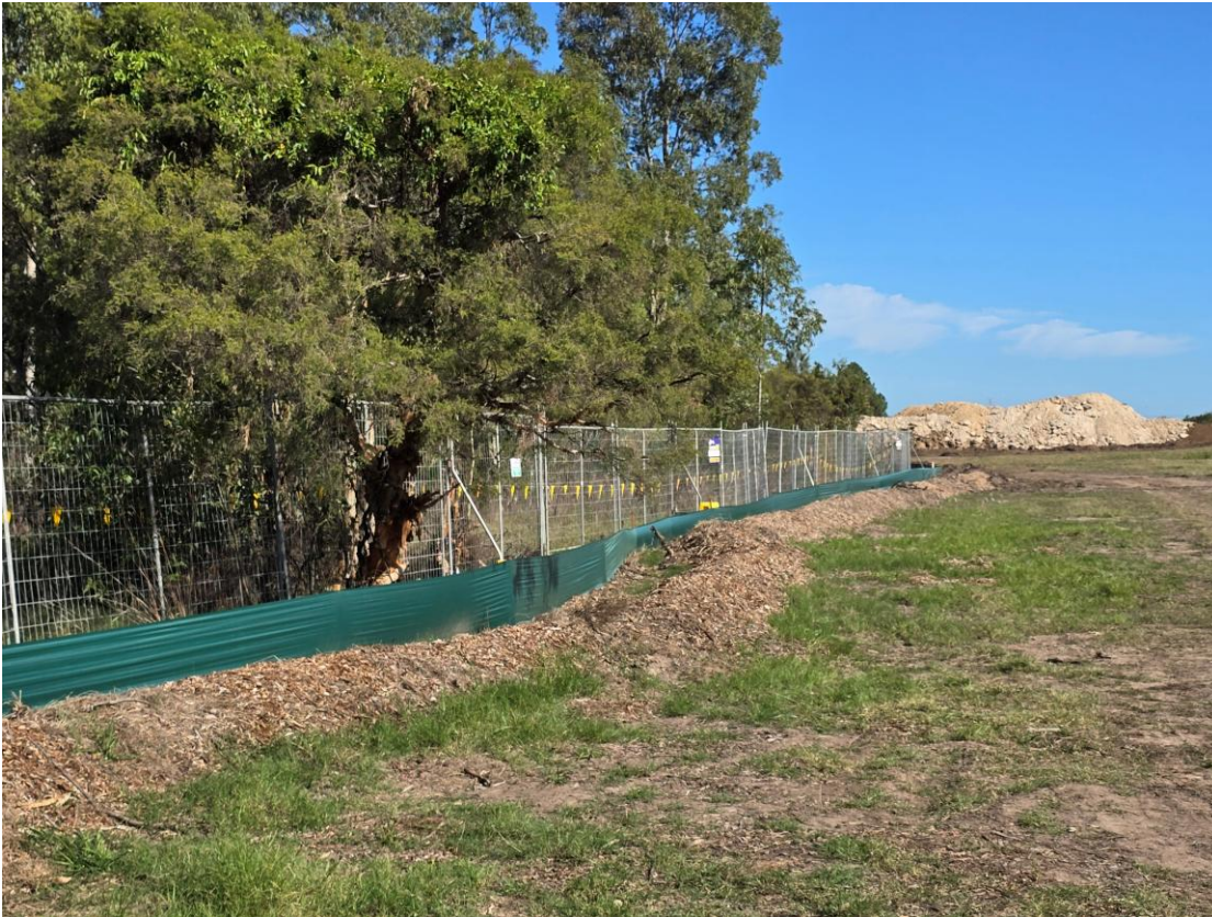
Plate 13 – ‘No Go’ fencing and signage with erosion and sediment controls
