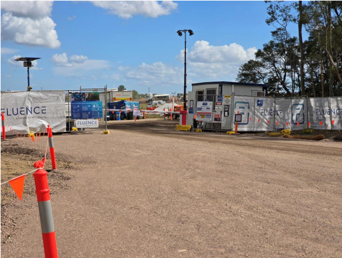
Plate 9 – Access road at security gate
