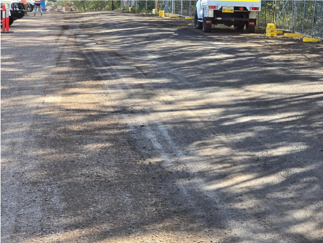
Plate 8 – Access road going to laydown areas
