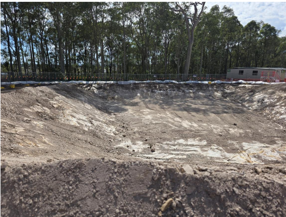
Plate 22 – Northern Water Basin being constructed
