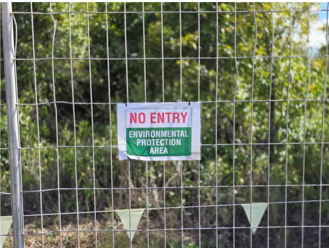
Plate 12 – 'No Go' signage in construction area
