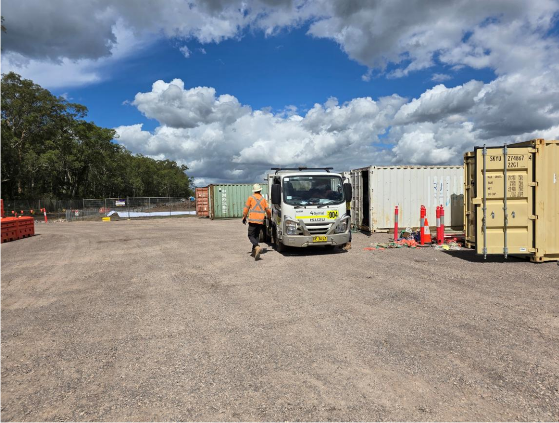
Plate 17 – Unloading and laydown area
