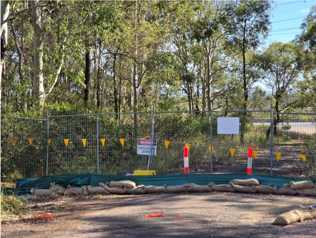
Plate 14 – ‘No Go’ fencing and signage with
