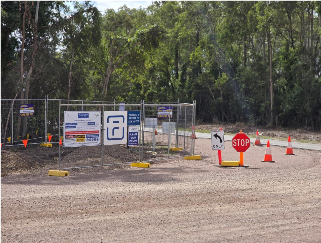
Plate 5 – Access point off Old Punt Road with traffic signage
