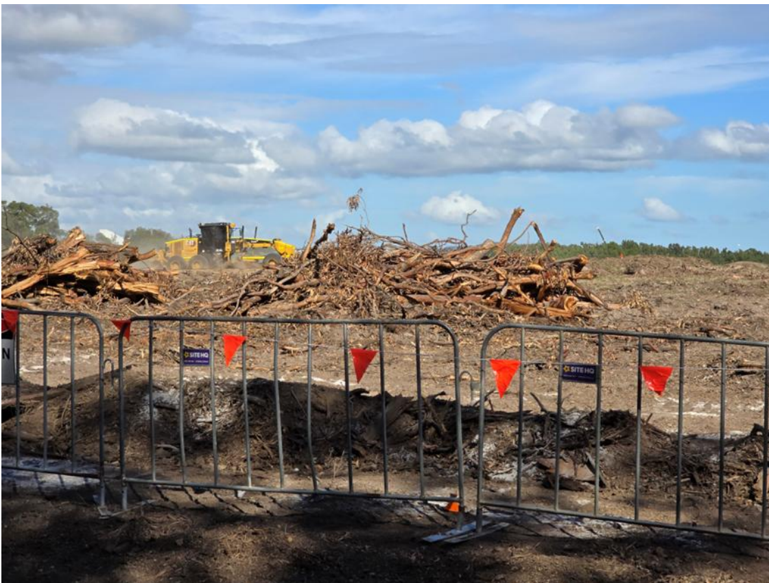
Plate 2 – Grader operating within the clearing and grubbing work area
