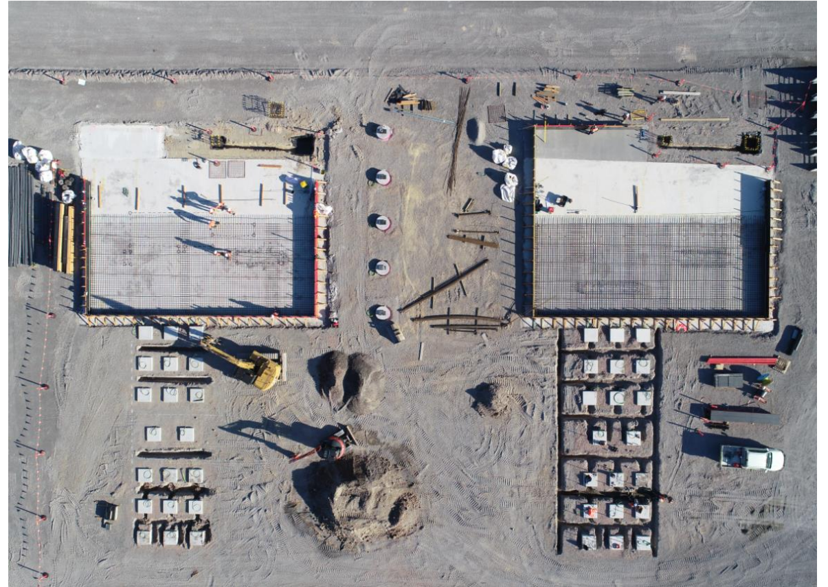
Footings and transformer bays for BESS substation
