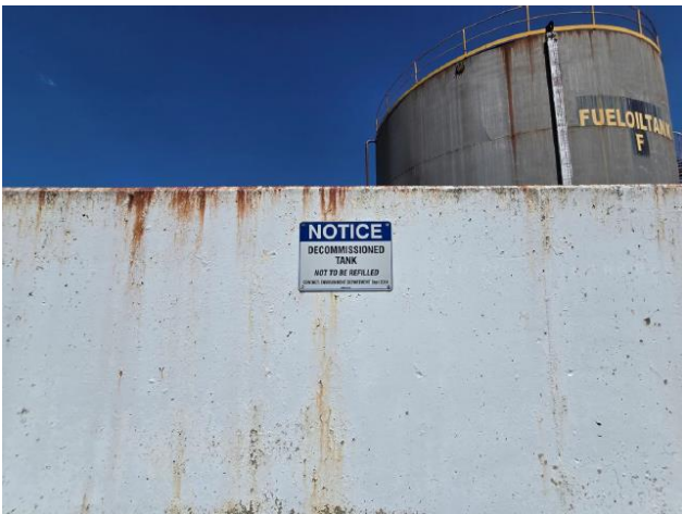
Photo 23 – Decommissioned bulk hydrocarbon storage tanks
