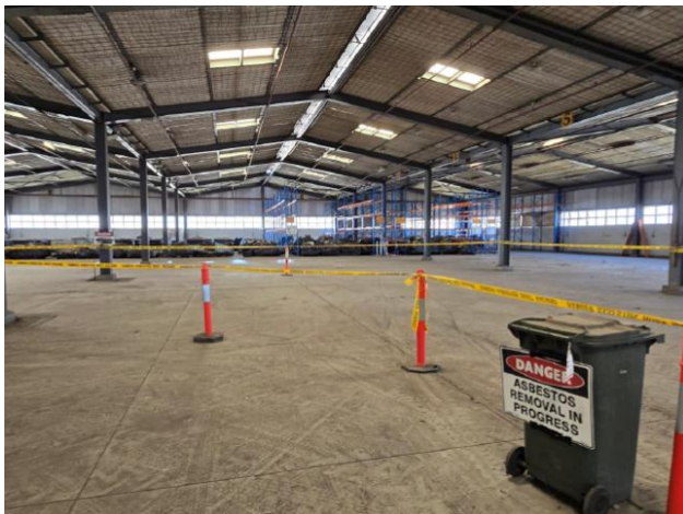
Photo 35 – Temporary asbestos storage facility at Liddell Power Station
