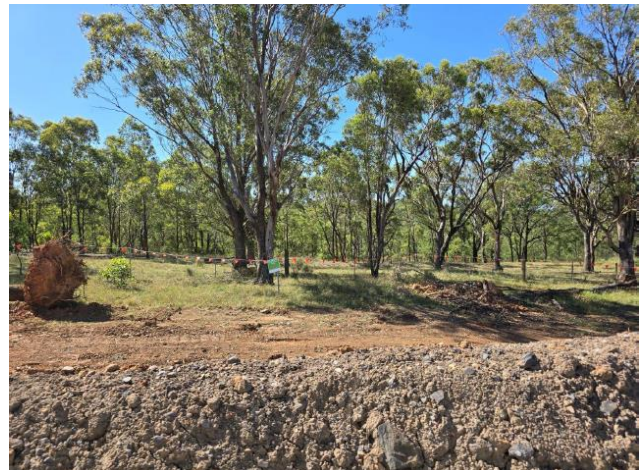
Photo 30 – 'No Go' zones demarcated around asbestos disposal facility and haul road construction area
