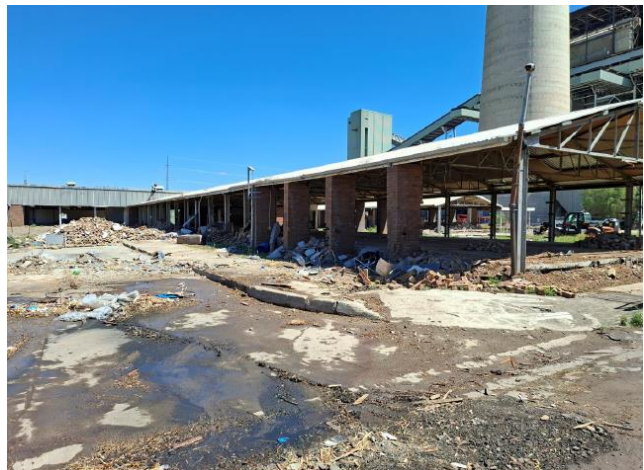
Photo 6 - Demolition area being kept watered down
