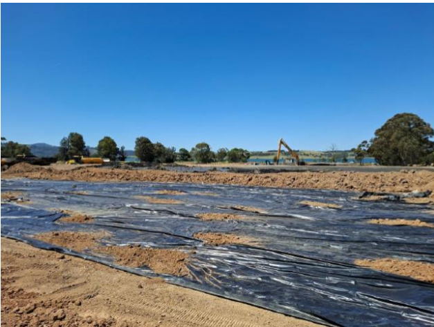
Photo 14 - Plastic lining for wet dump used for desilting sludge from oil and grit trap material
