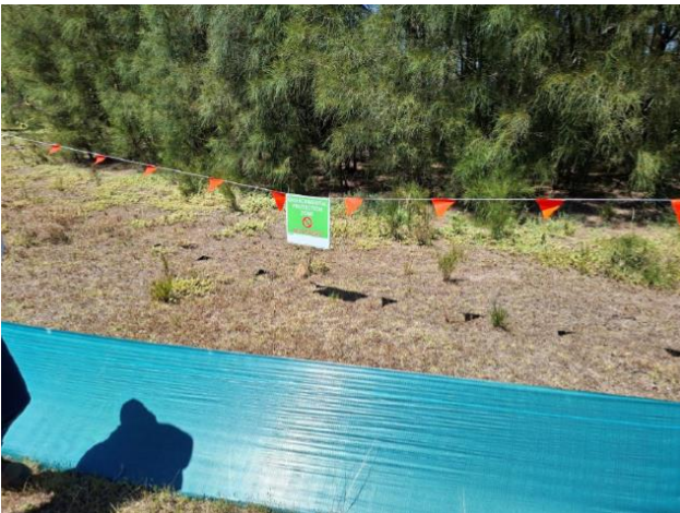
Photo 29 – Frog exclusion fencing and 'No Go' zones demarcated at Liddell Power Station oil and grit trap works area
