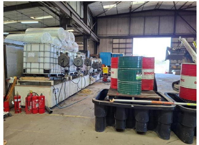
Photo 15 - Bunded chemicals and fire fighting equipment in store area of Liddell Power Station
