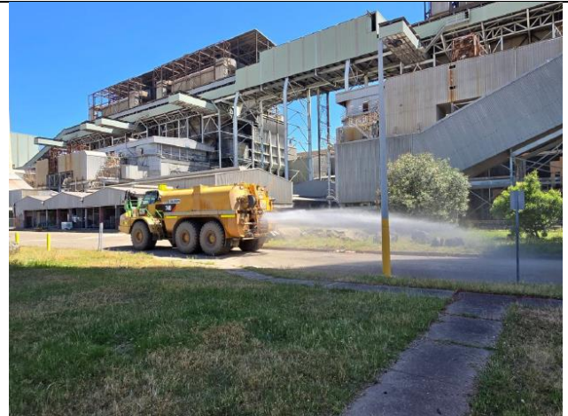
Photo 4 - Watercart in operation around the Liddell Power Station demolition works area
