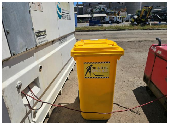
Photo 18 - Spill kit next to fuel storage tank
