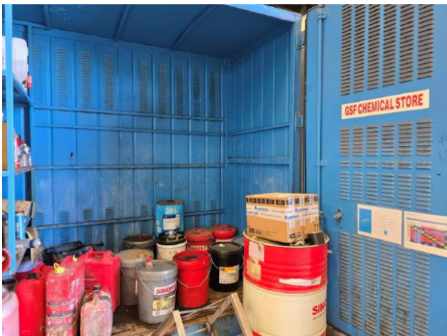
Photo 16 - Self-bunded chemical storage area at Liddell Power Station
