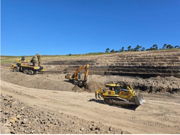
Photo 1 - Asbestos disposal facility currently under construction
