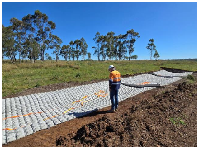
Photo 12 - Geofabric lining for drains to exclude clean water from asbestos disposal facility
