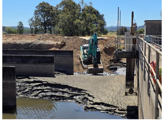
Photo 2 - Excavator desilting the Liddell oil and grit trap within Stage 1 works area
