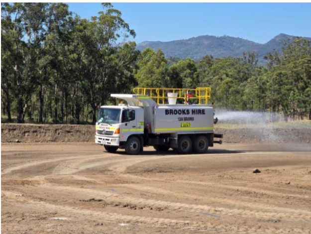
Photo 5 - Watercart in operation around the asbestos disposal facility construction works
