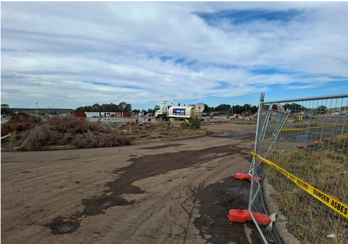
Plate 28 –Water Cart available at the Liddell demolition area
