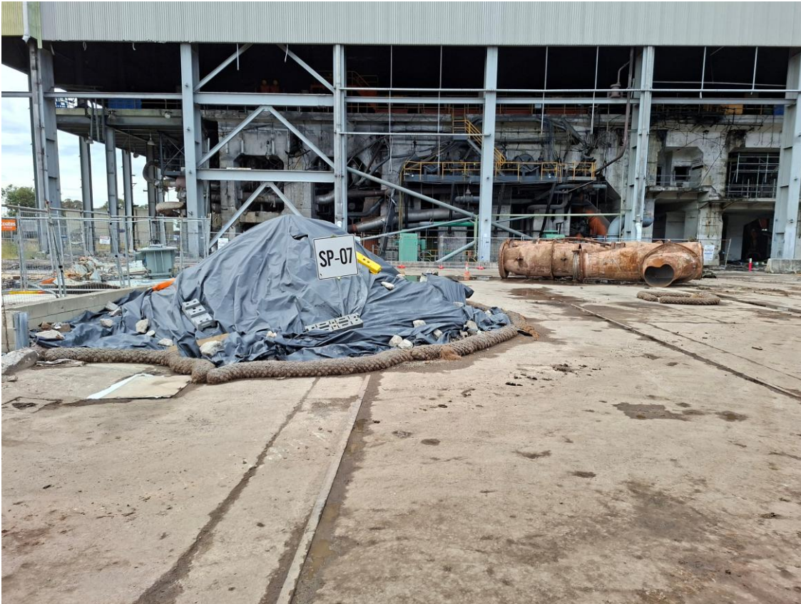
Plate 31 Example of covered stockpile to prevent dust
