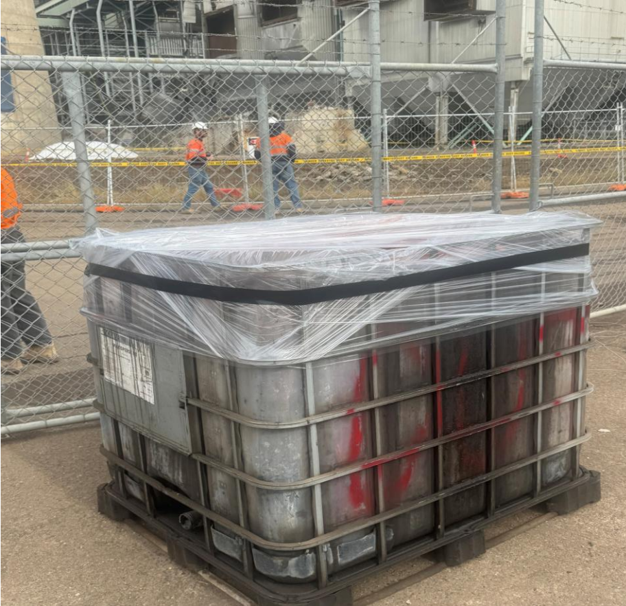
Plate 9 – Tub filled with separated Copper at the Liddell demolition area
