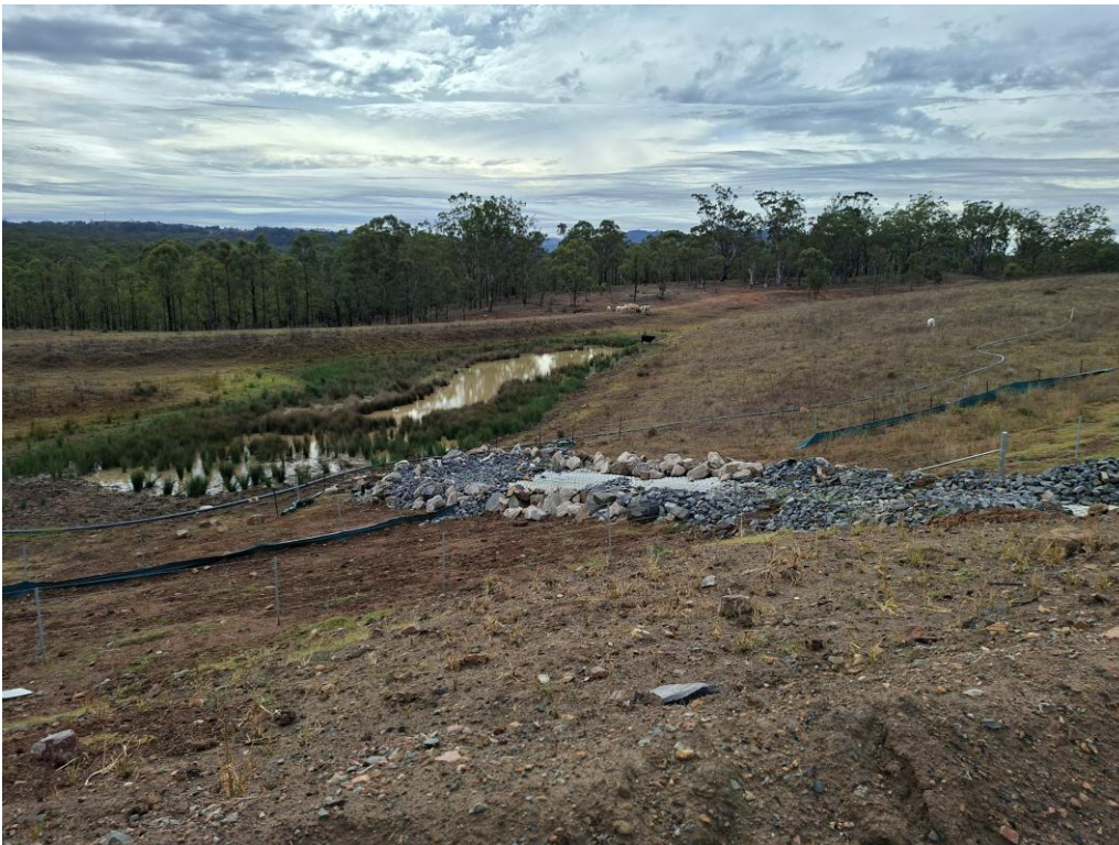
Plate 6 – Sediment control drains and dam downslope of the asbestos disposal facility
