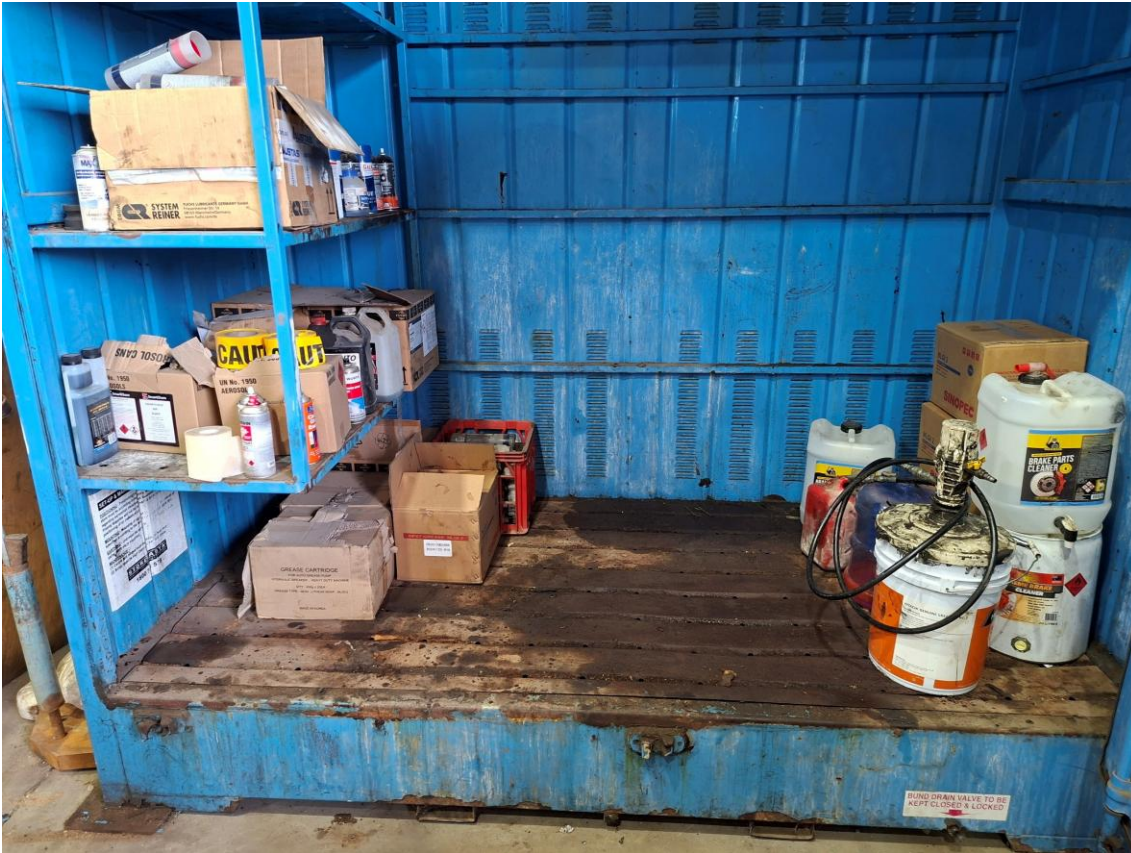
Plate 11 – Self-bunded chemical storage area at Liddell demolition area
