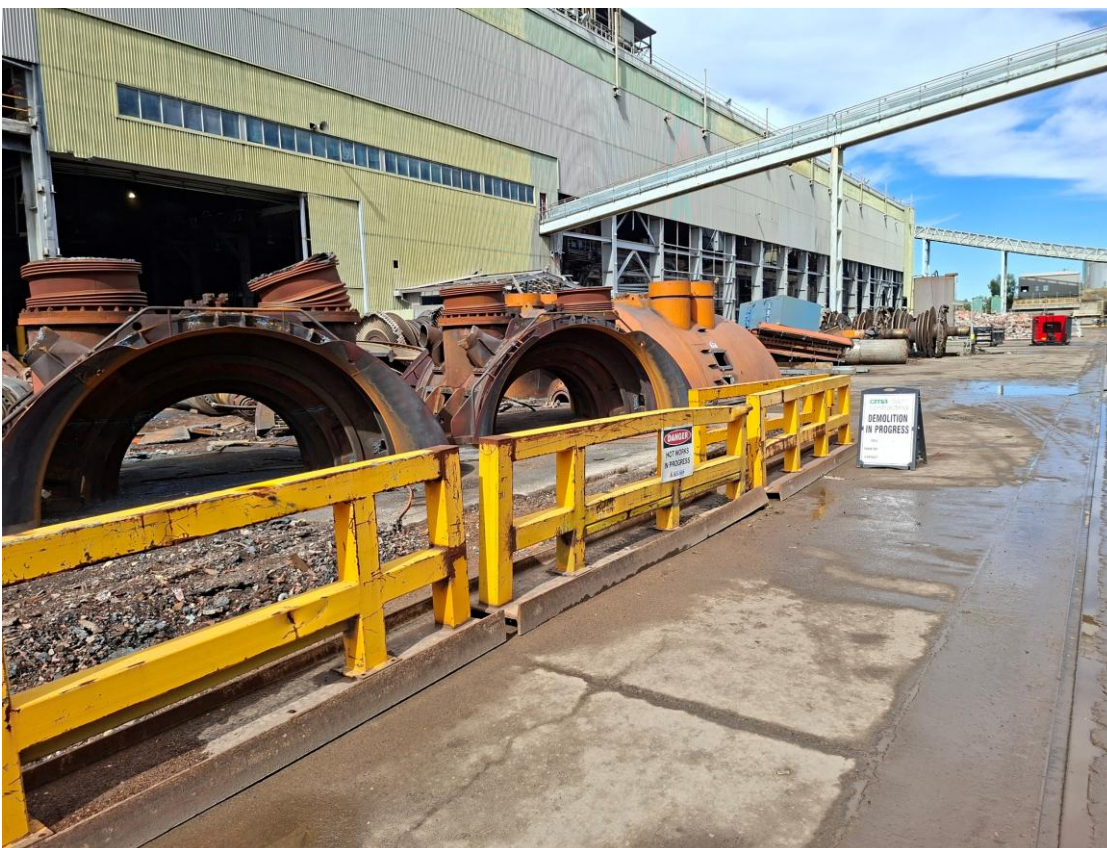
Plate 32 – Segregated metal waste at the Liddell demolition area
