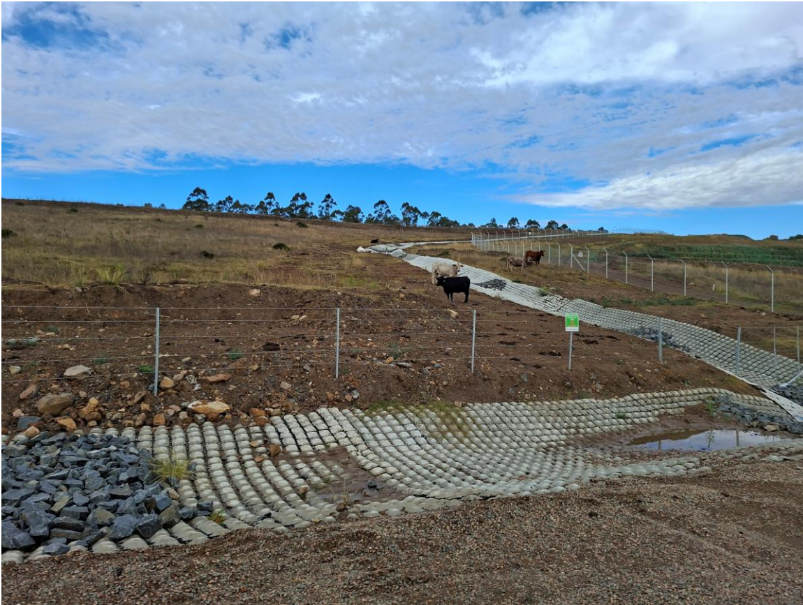
Plate 3– Fenced boundary of the Project area and concrete matting in diversion drains
