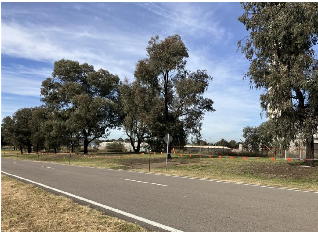
Plate 22 – 'No Go' zones demarcated around vegetation adjacent to Liddell demolition area
