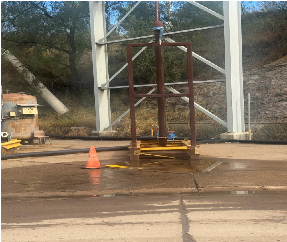
Plate 5 – Fill point in place near the Liddell demolition area
