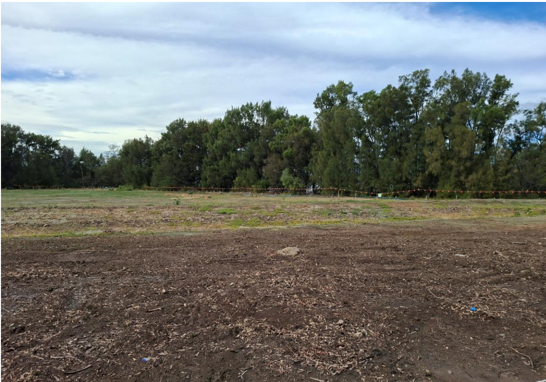
Plate 26 – “No go” fencing to protect sensitive environmental areas around the Liddell demolition area boundary
