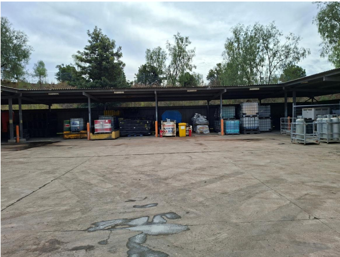
Plate 30 – Waste segregation and control at the Liddell demolition area
