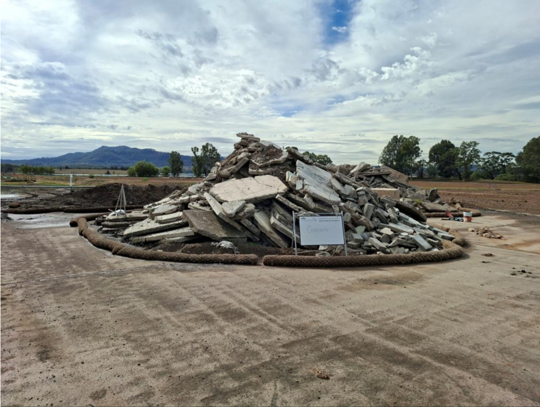
Plate 7 – Concrete stockpiling at the Liddell demolition area
