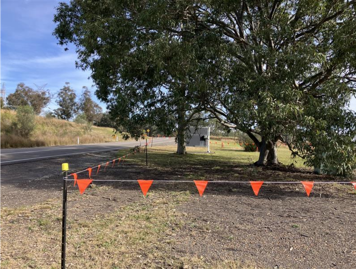
Plate 23 – ‘No Go’ zones demarcated around vegetation adjacent to Liddell demolition area
