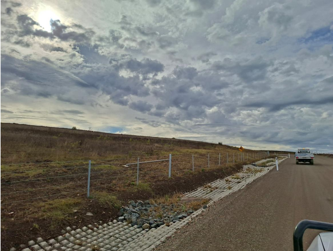
Plate 25 – Fencing and concrete matting along access road to asbestos disposal facility
