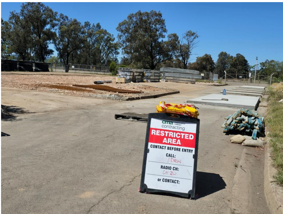
Plate 20 – Demarcation of restricted area in the Liddell demolition area
