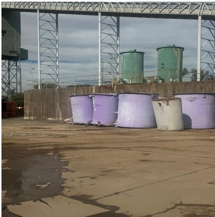
Plate 15 – Decommissioned bulk hydrocarbon storage tanks at the Liddell demolition area
