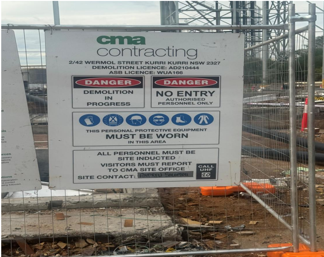
Plate 19 – Safety signage at the entry to the Liddell demolition work area
