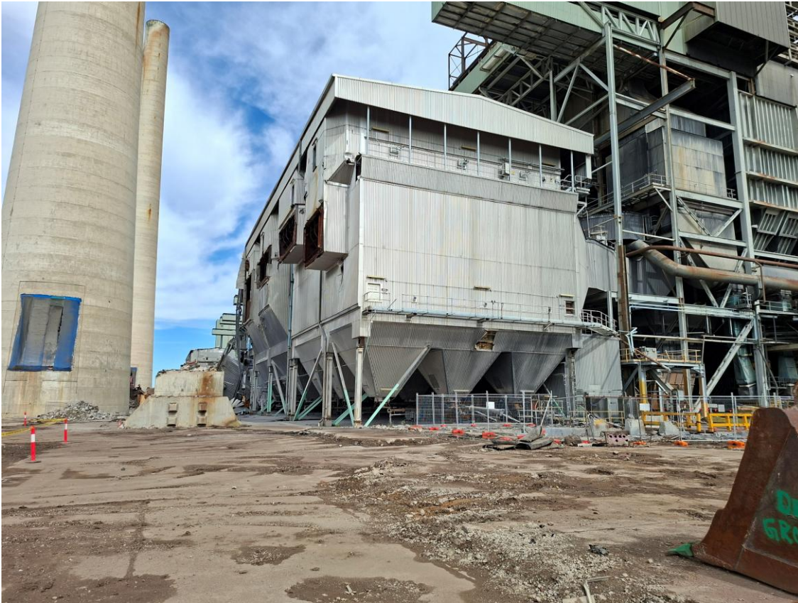
Plate 29 – Active demolition area at the Liddell site
