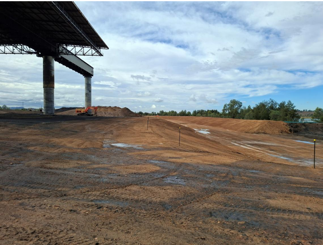
Plate 10 – Drainage structure construction near the Coal Handling Plant demolition area
