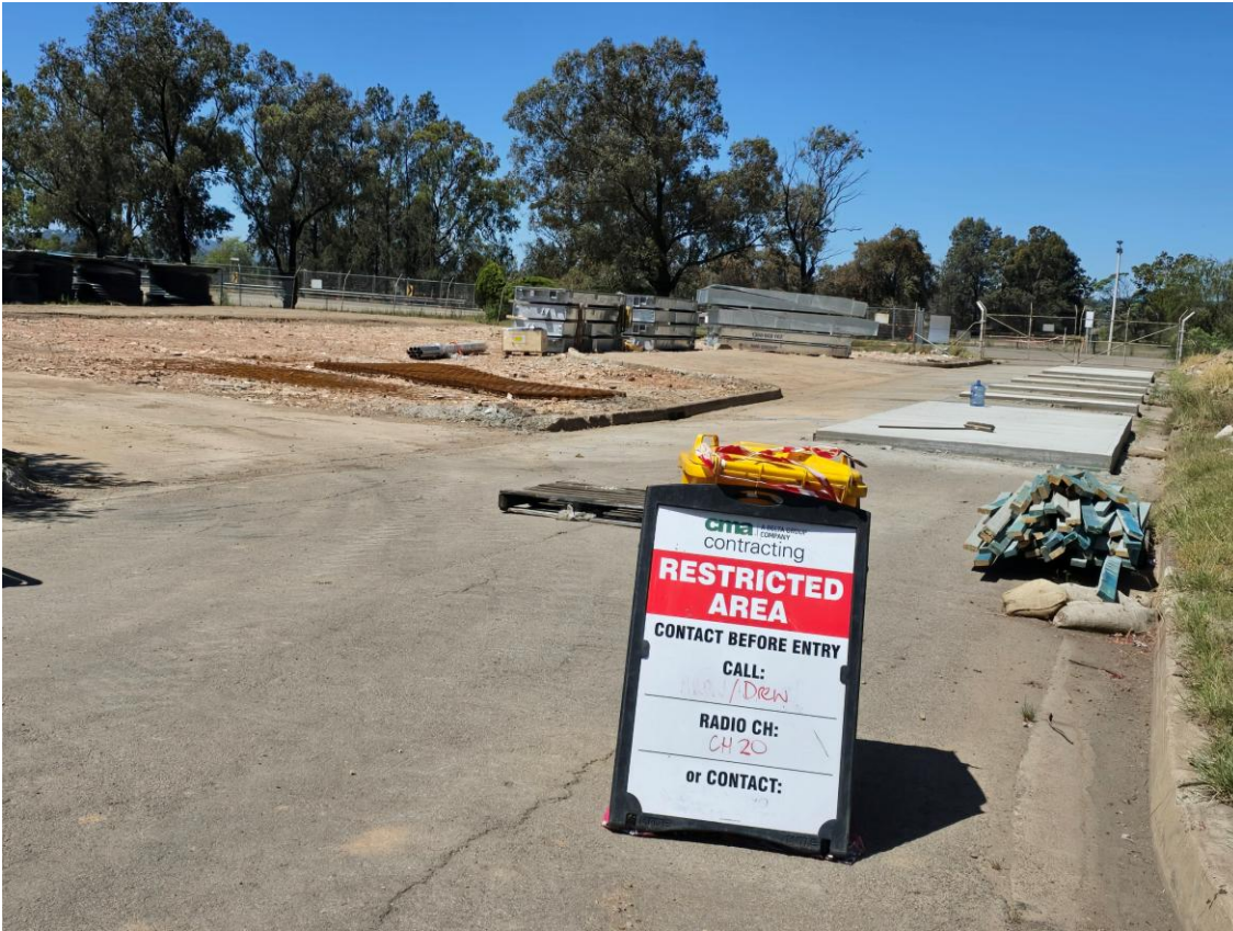
Plate 33 – Demarcation of restricted area in demolition work area
