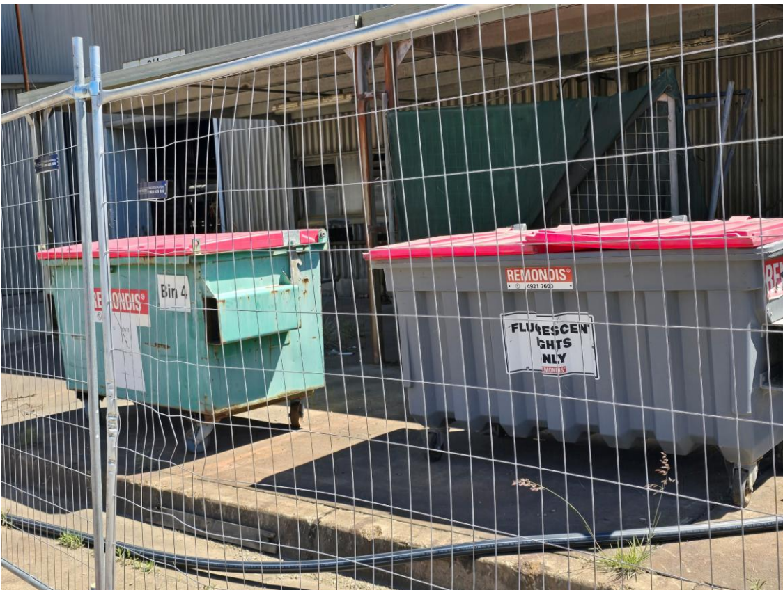
Plate 28 – Waste segregation at Liddell Power Station demolition area
