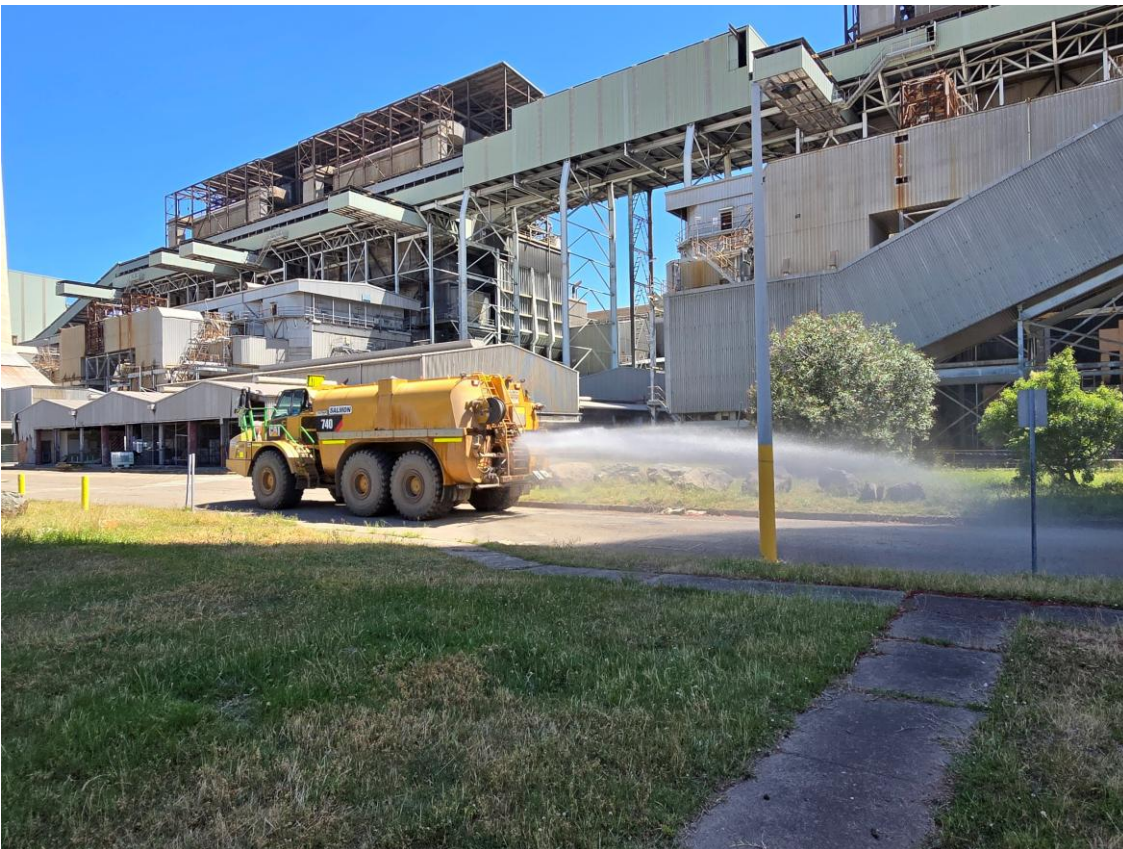
Plate 4 – Watercart in operation around the Liddell Power Station demolition works area
