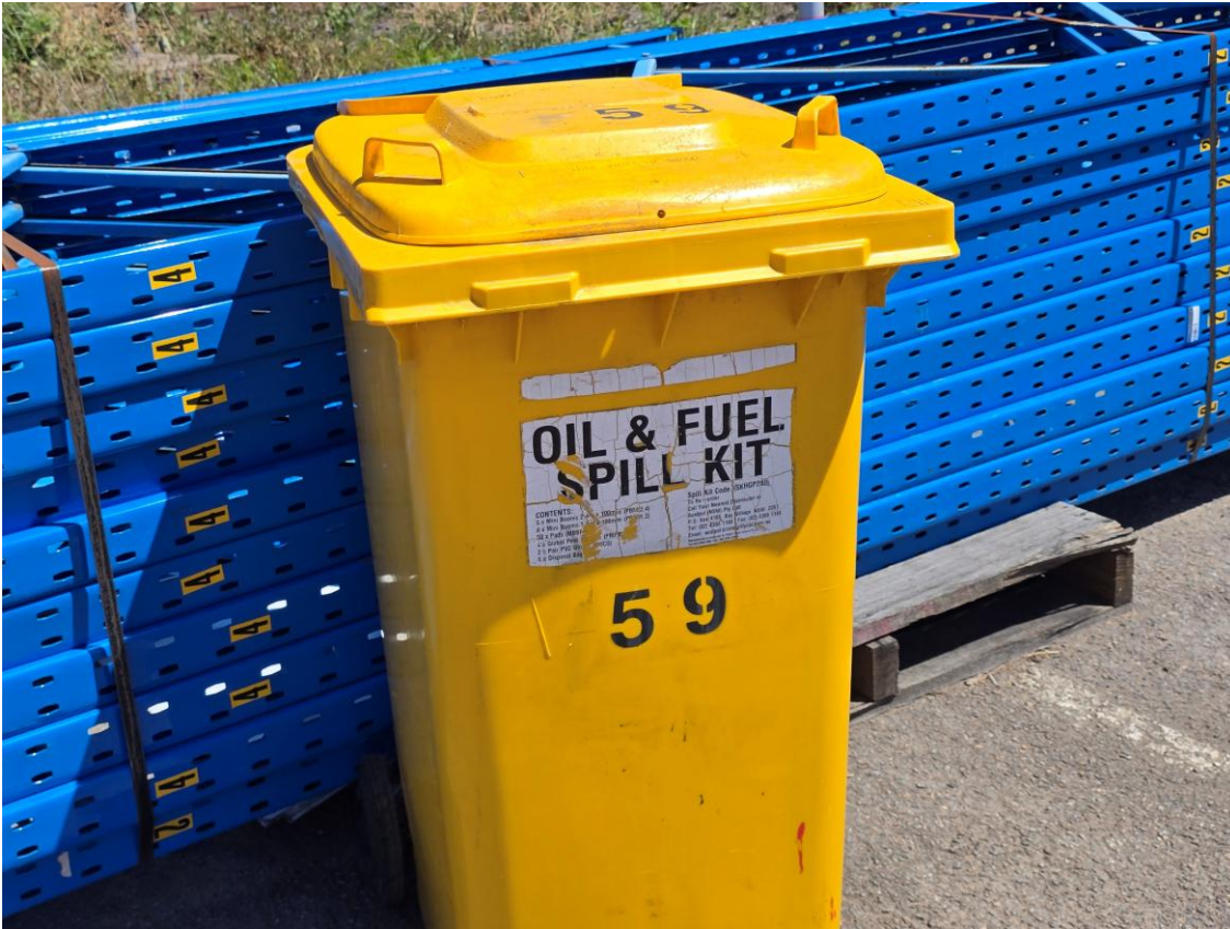
Plate 19 – Spill kit in Liddell Power Station demolition work area
