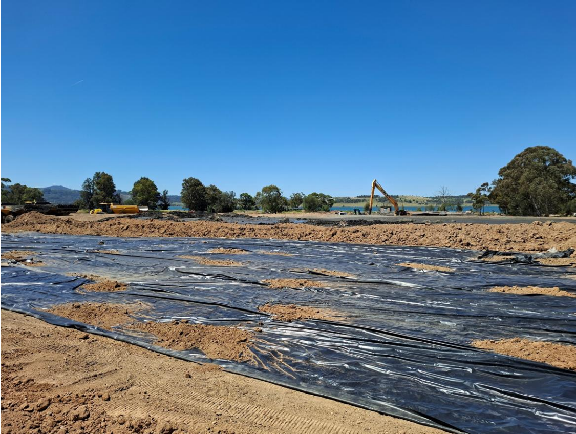
Plate 15 – Plastic lining for wet dump used for desilting sludge from oil and grit trap material
