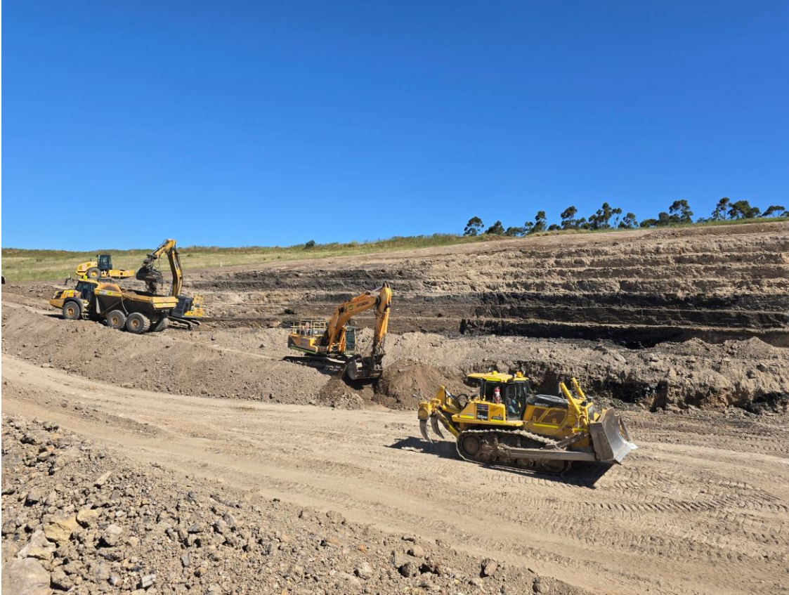
Plate 1 - Asbestos disposal facility currently under construction
