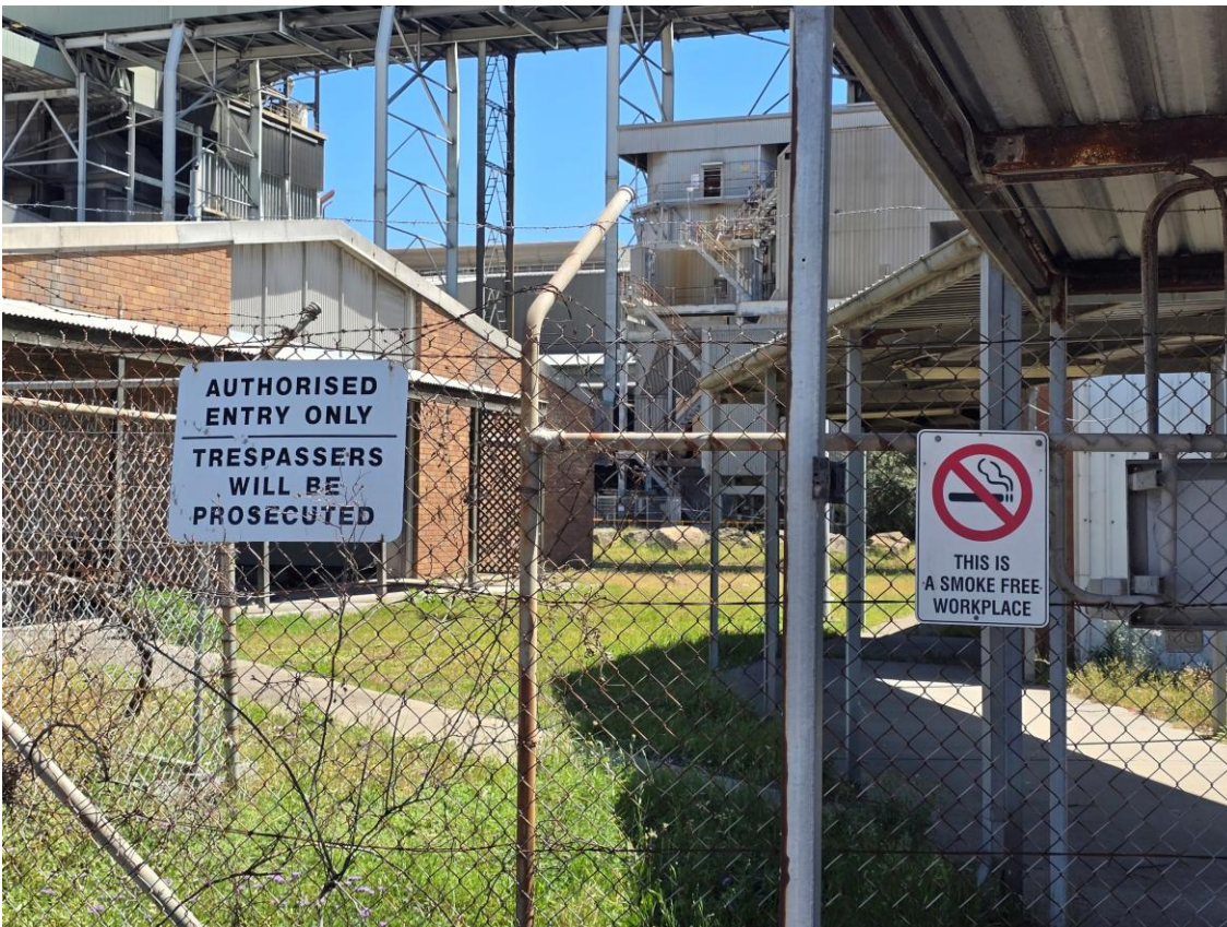
Plate 32 – Safety signage going into demolition work area
