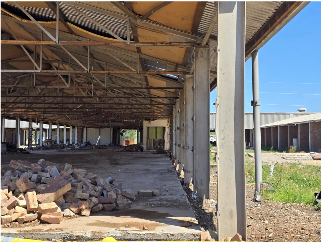
Plate 34 – Stripping out demolition works at Liddell Power Station
