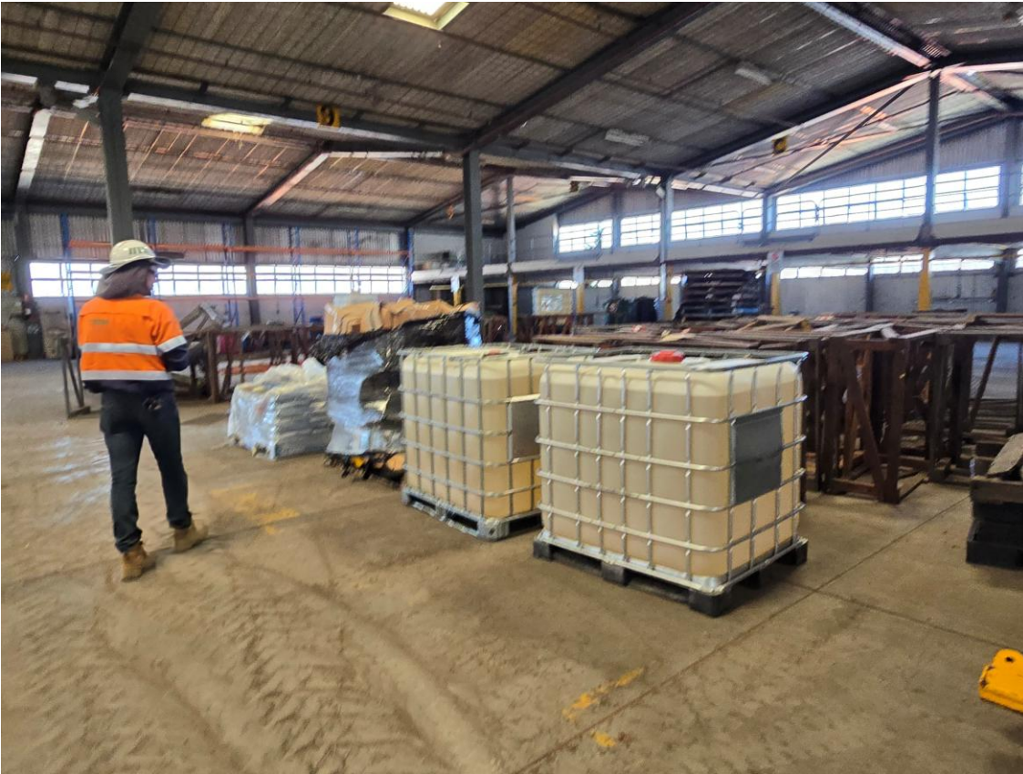
Plate 21 – Spill kit in Liddell Power Station demolition work area
