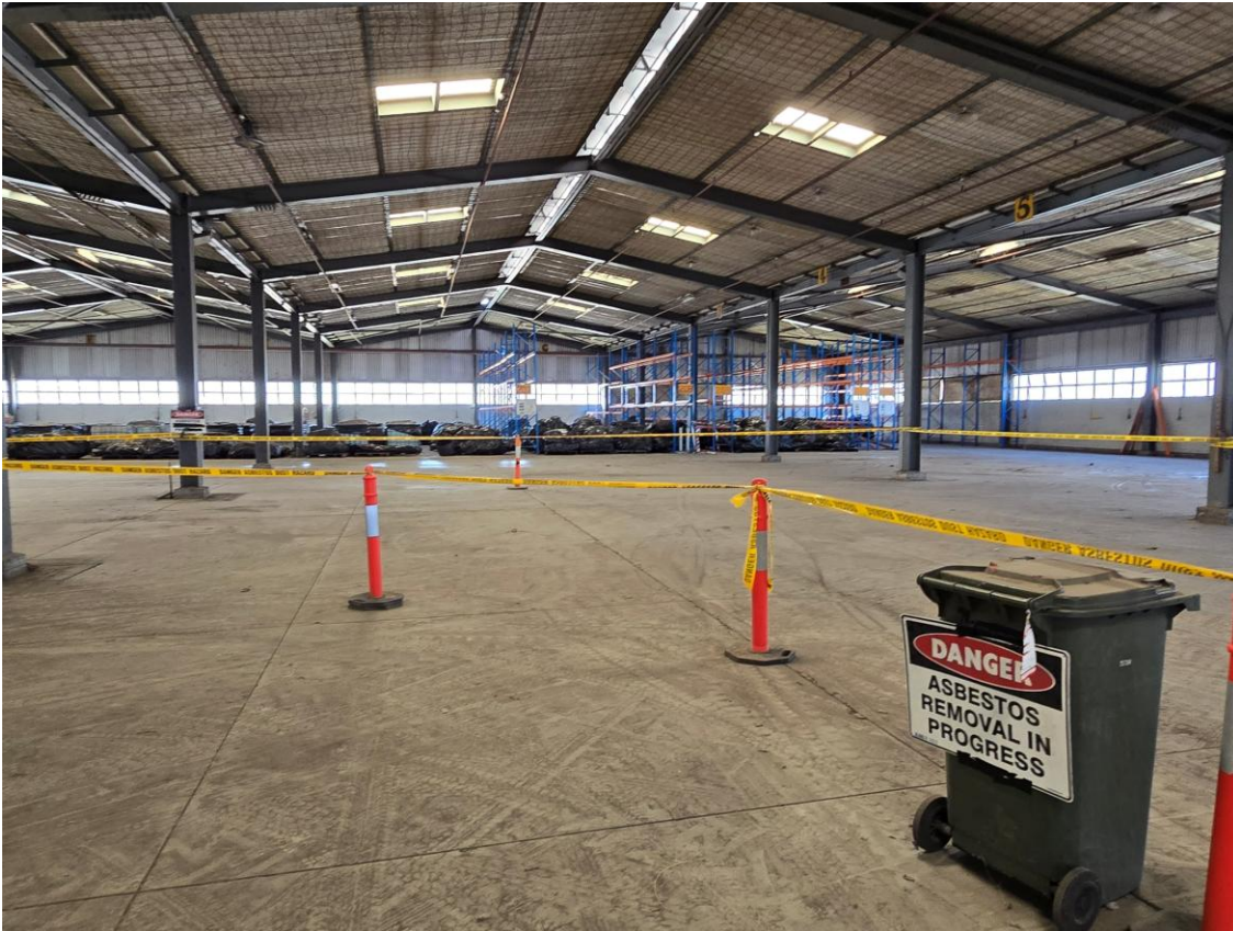
Plate 35 – Temporary asbestos storage facility at Liddell Power Station
