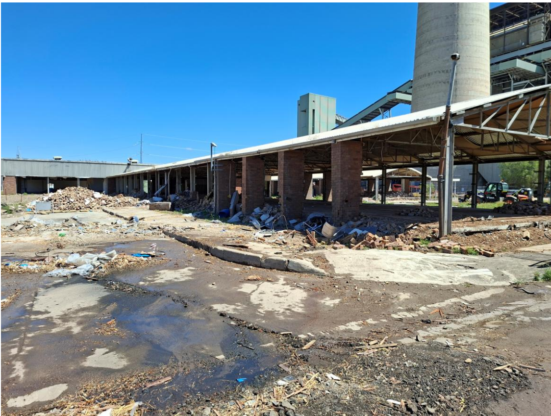
Plate 6 – Demolition area being kept watered down
