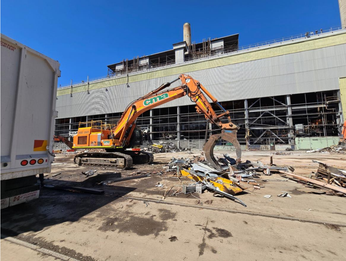
Plate 3 - Demolition stripping out works occurring at the Liddell Power Station
