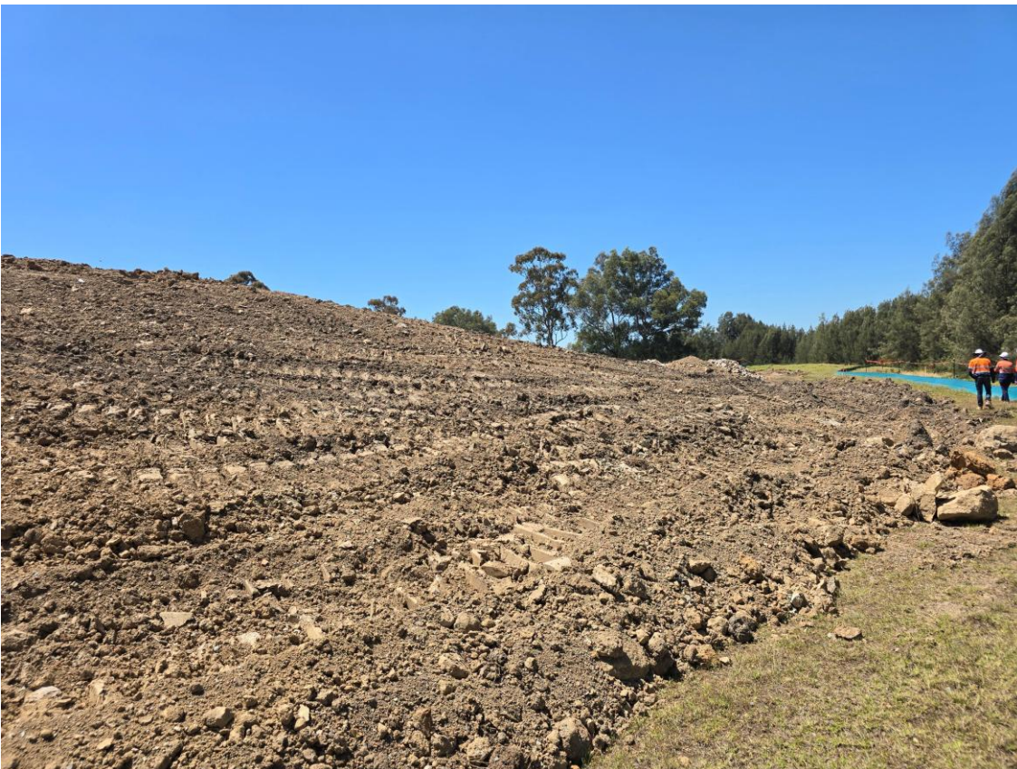
Plate 8 – Stockpiles within Stage 1 works area being shaped in preparation for hydroseeding
