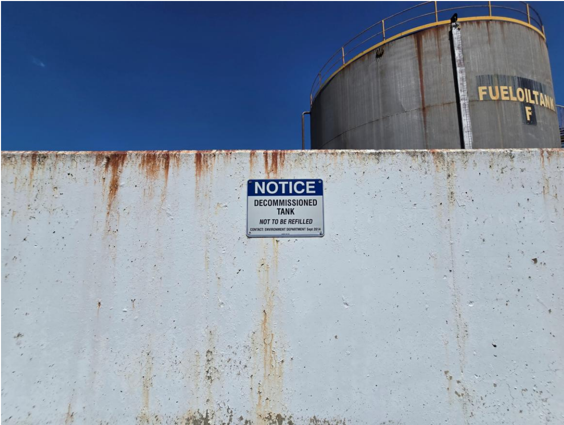
Plate 23 – Decommissioned bulk hydrocarbon storage tanks
