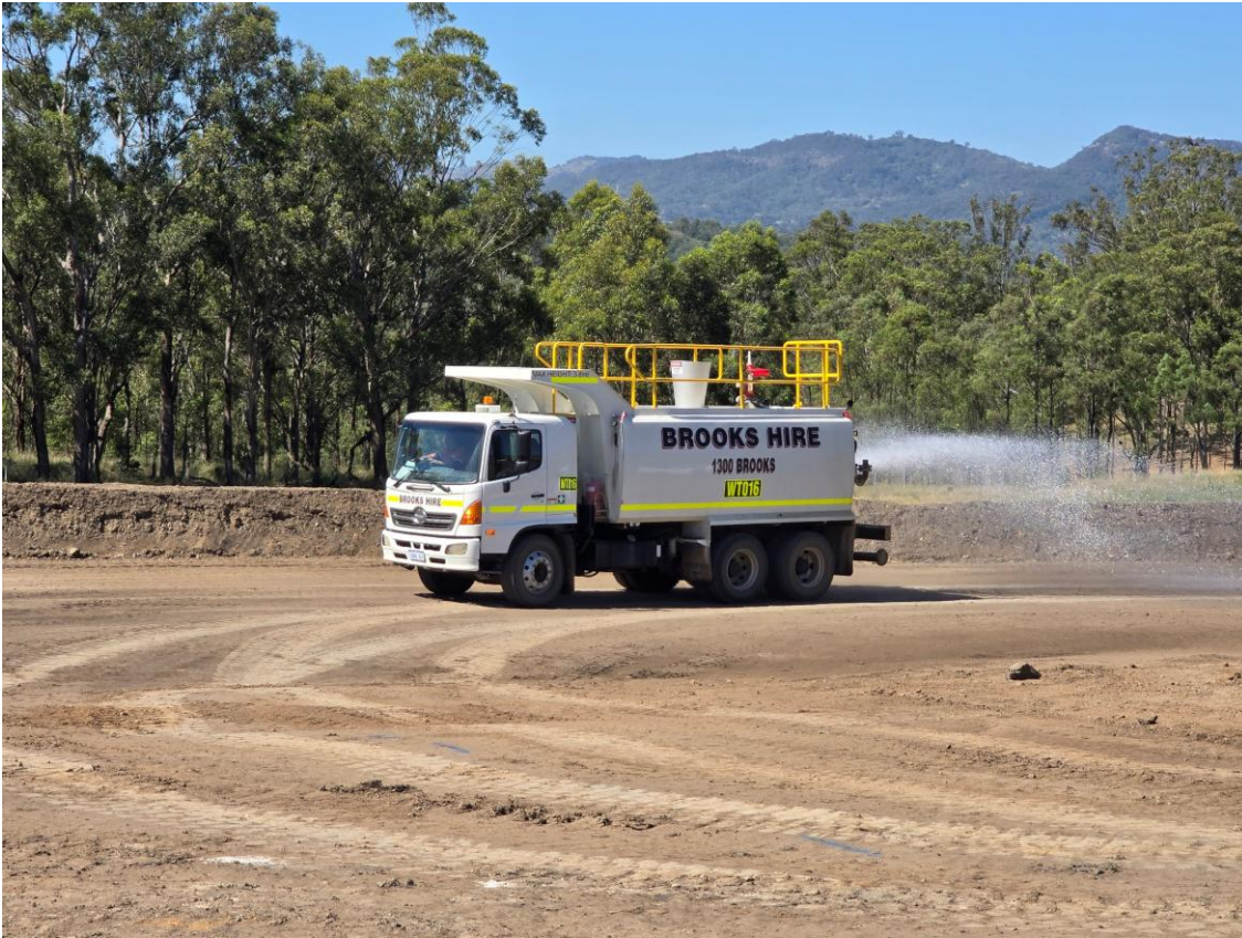
Plate 5 – Watercart in operation around the asbestos disposal facility construction works
