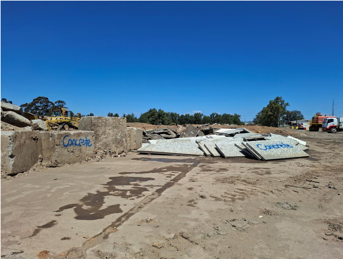
Plate 9 – Concrete stockpiling for reuse
