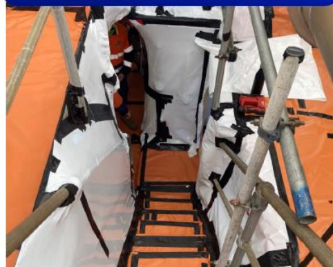
Steam pipe prior to ACM removal
