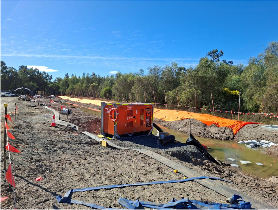
Plate 20 – Pump on drain for Stage 2 work area
