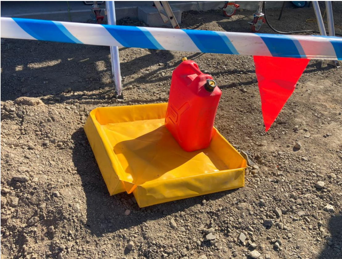
Plate 3 - Bunded storage for small volumes of hazardous chemicals at Stage 2
