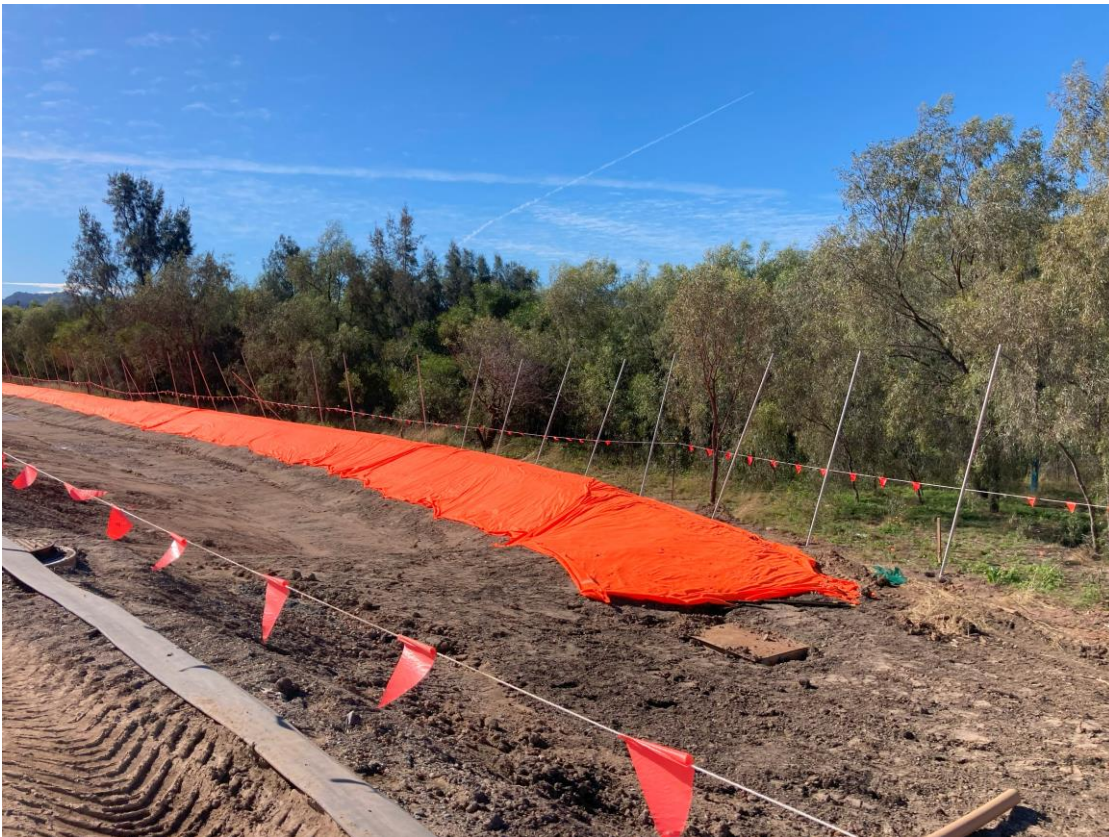
Plate 12 – Installation of permanent fence within perimeter of Stage 2 disturbance boundary
