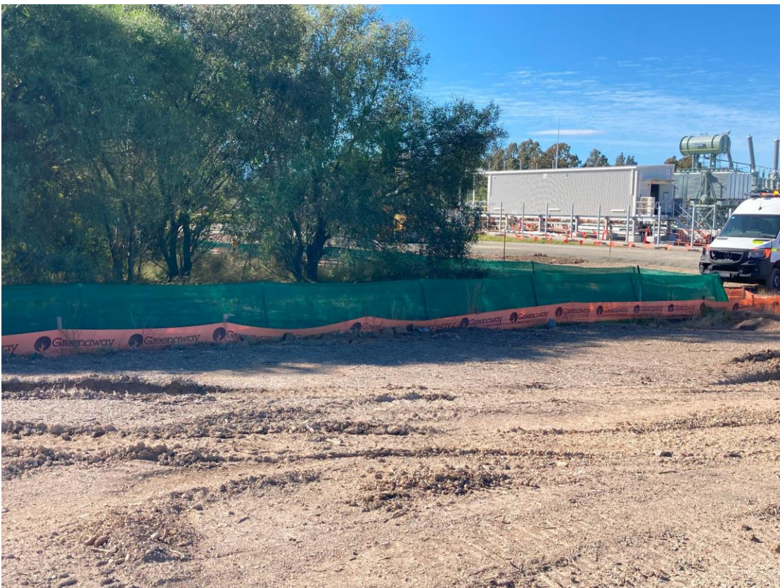
Plate 21 – Sediment controls in place
