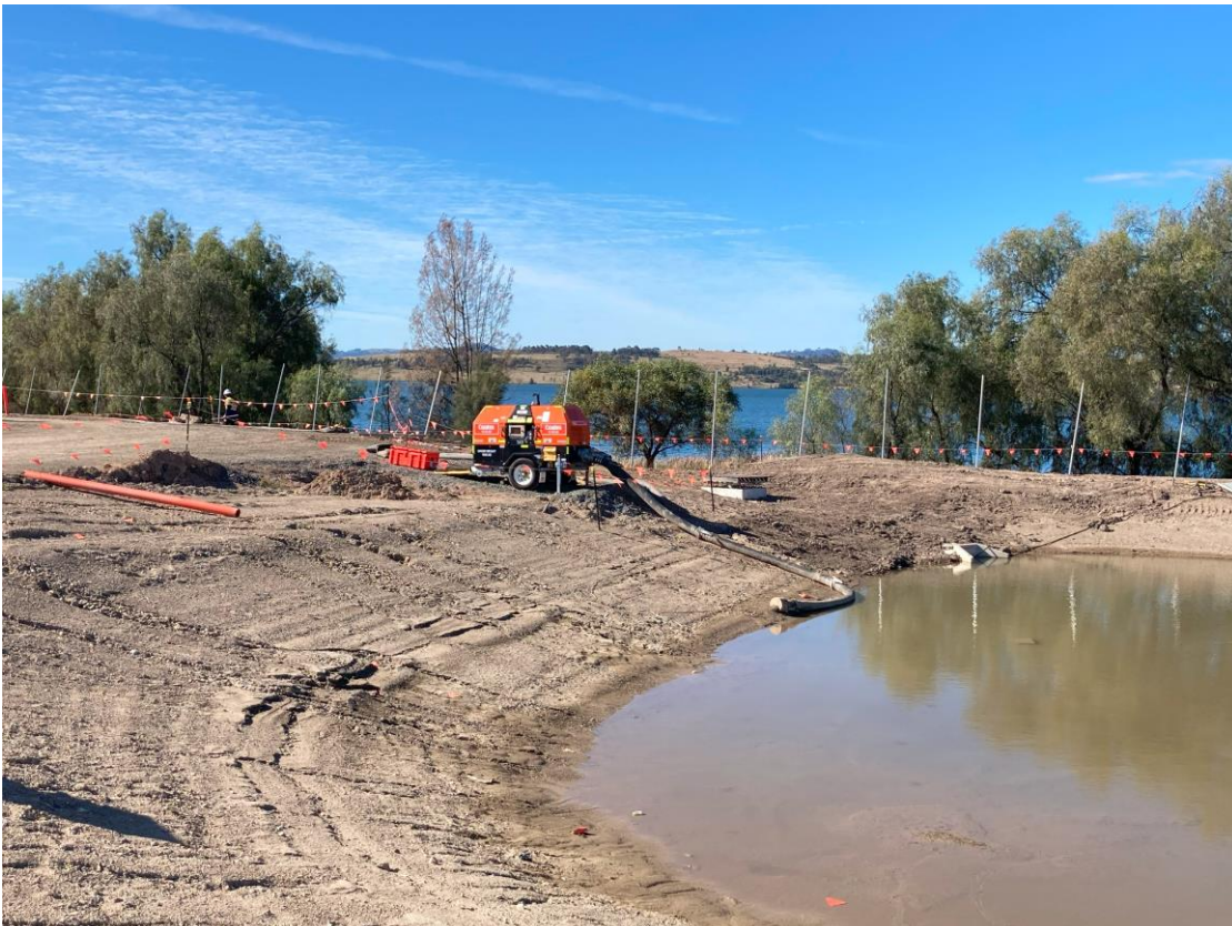
Plate 19 – Pump on sediment dam for Stage 2 work area
