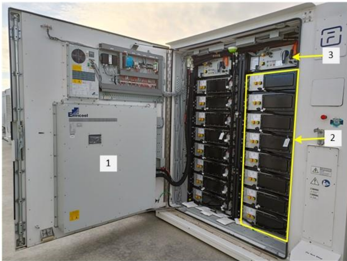
Plate 2: Fluence Cube: internal view
