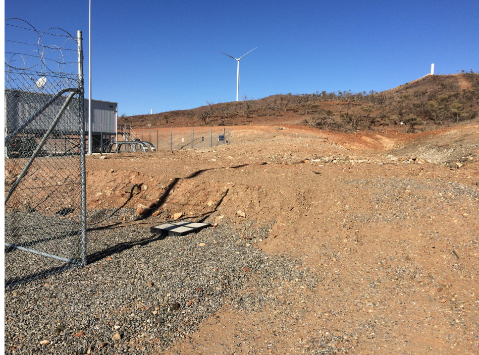
Item 2 – Rehabilitation of area behind 33kv substation (GE Catcon area) not undertaken. Topsoil dressing and contour ripping of area required as a priority due to exposed area adjacent to realigned watercourse posing a erosion risk.
