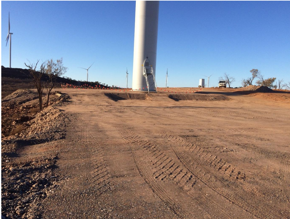
T23 proofed rolled and ready for punch listing
