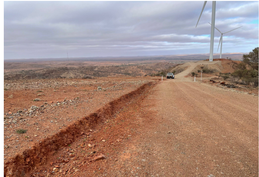
Photo C4: Access Road – Road Verge Drainage Controls
