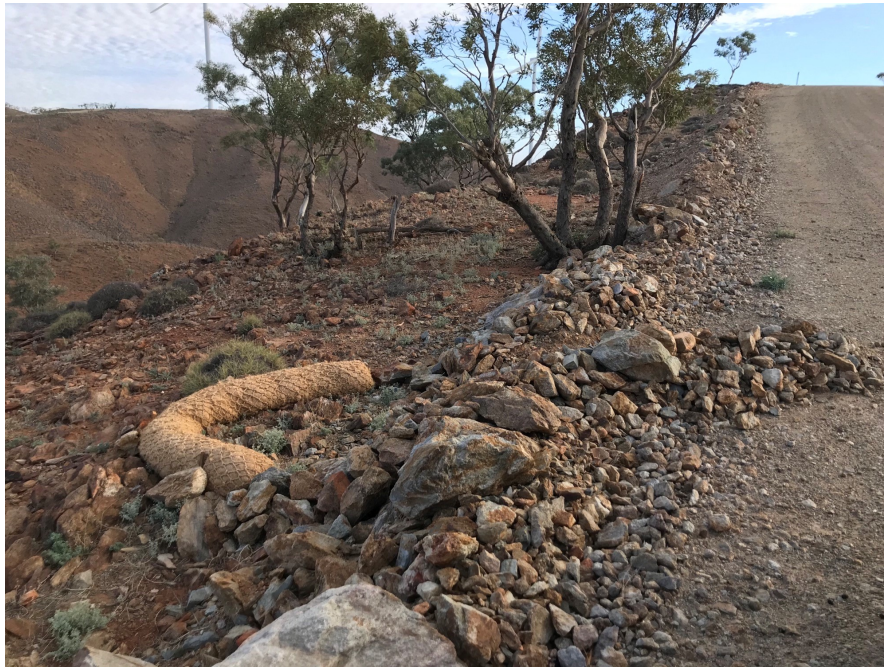
Photo C9: Area 7 – Example of a Rock Cross-Bank with Outlet Protection (coir log)
