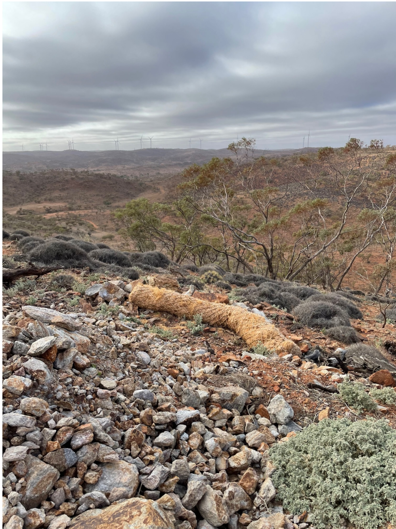
Photo C7: Area 7 – Example of a Rock Cross-Bank with Outlet Protection (coir log)
