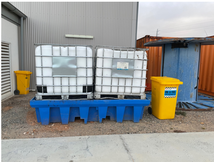
Photo C1: Operations and Maintenance Facility – Bunded Waste Oil Storage
