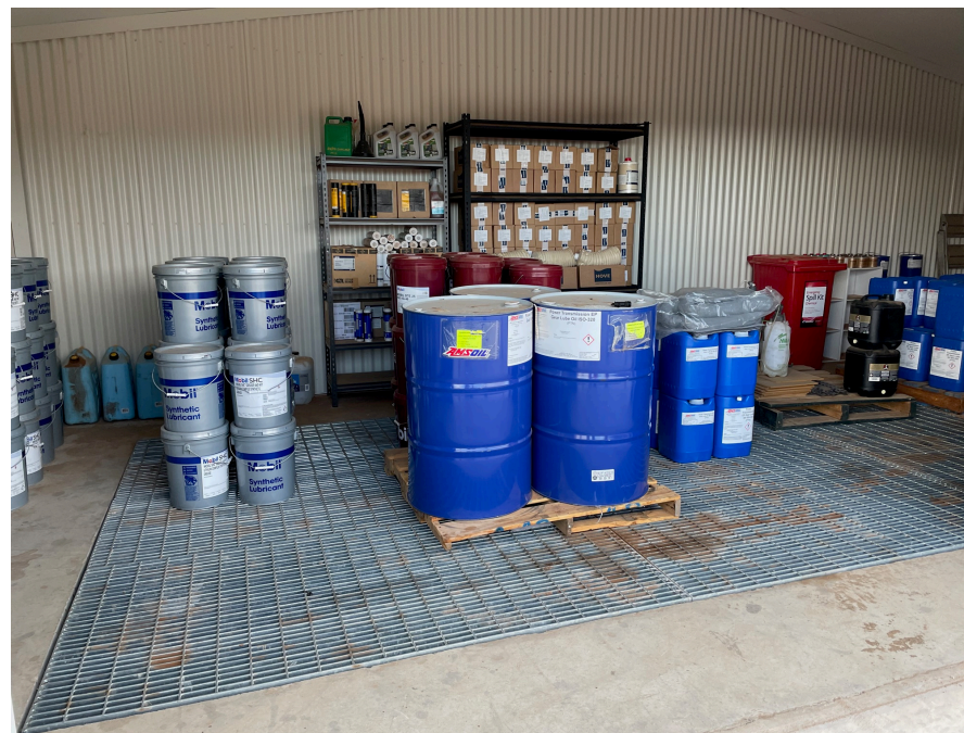
Photo C2: Operations and Maintenance Facility – Bunded Chemical Storage
