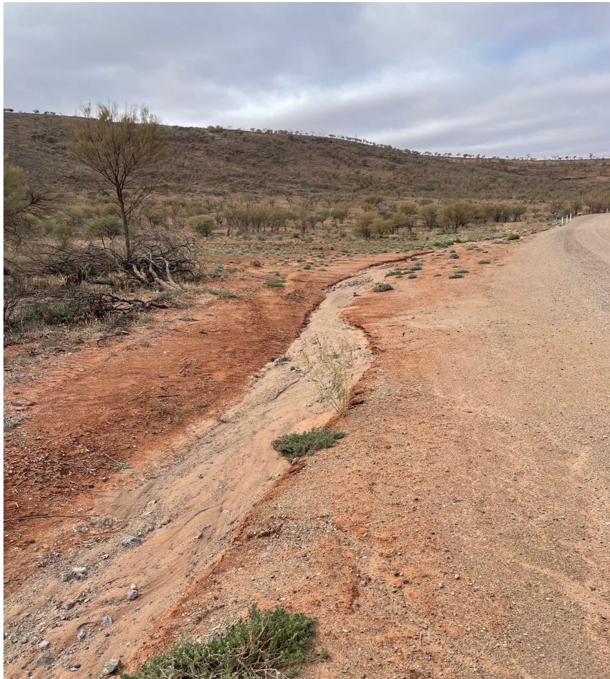
Photo C11: Roadside Erosion (South of Operations and Maintenance Building)
