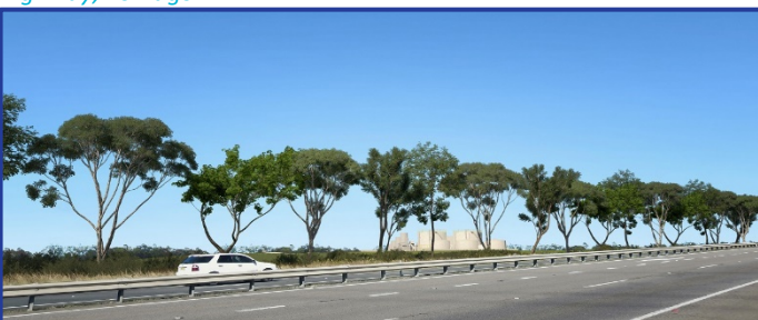
Figure 2: Gas turbine technology as seen from Pacific Highway, Tomago.
