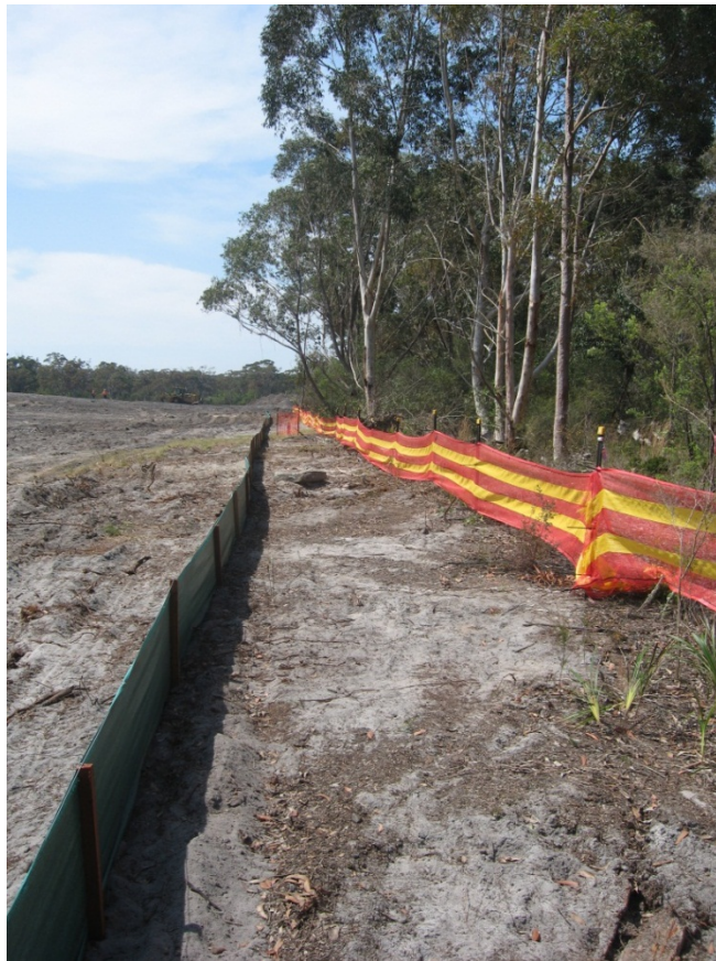
Figure 4.1 Silt fencing and parawebbing installed along Site Boundary
