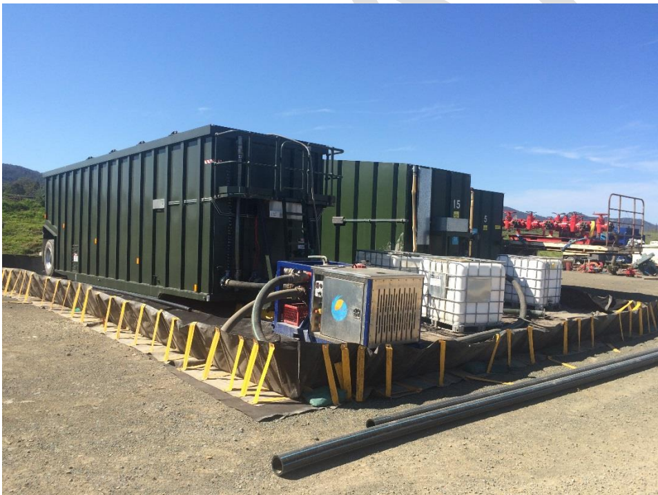
Water management facility with bunding used to support the workover rig.
