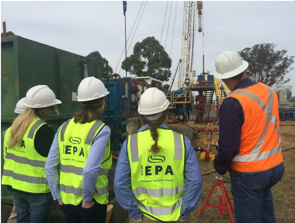
EPA Gas Regulation Branch site inspection of the Workover Rig during the Plug and Abandonment works.
