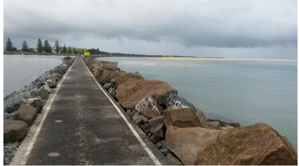
Photo 4 – MR01 – Breakwall at Harrington
