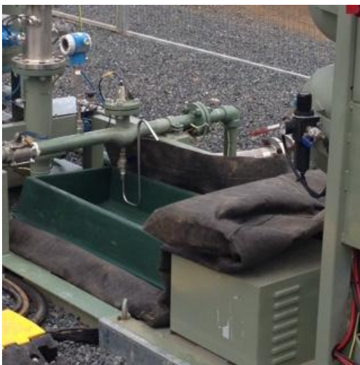
Figure 2 - Swagelok stainless steel sampling spout with primary and secondary containment in place.
