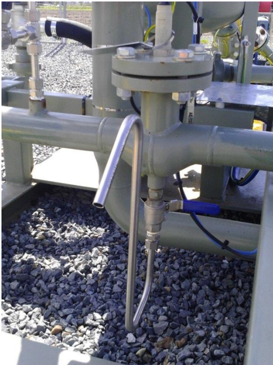
Figure 1 - Swagelok stainless steel sampling spout (detachable)
