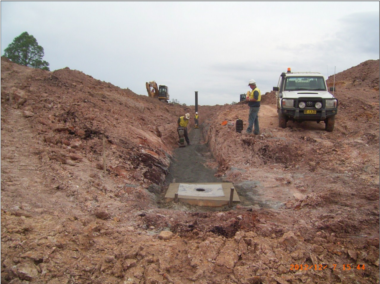
A 1 metre concrete apron surrounds the pipe inlet.
