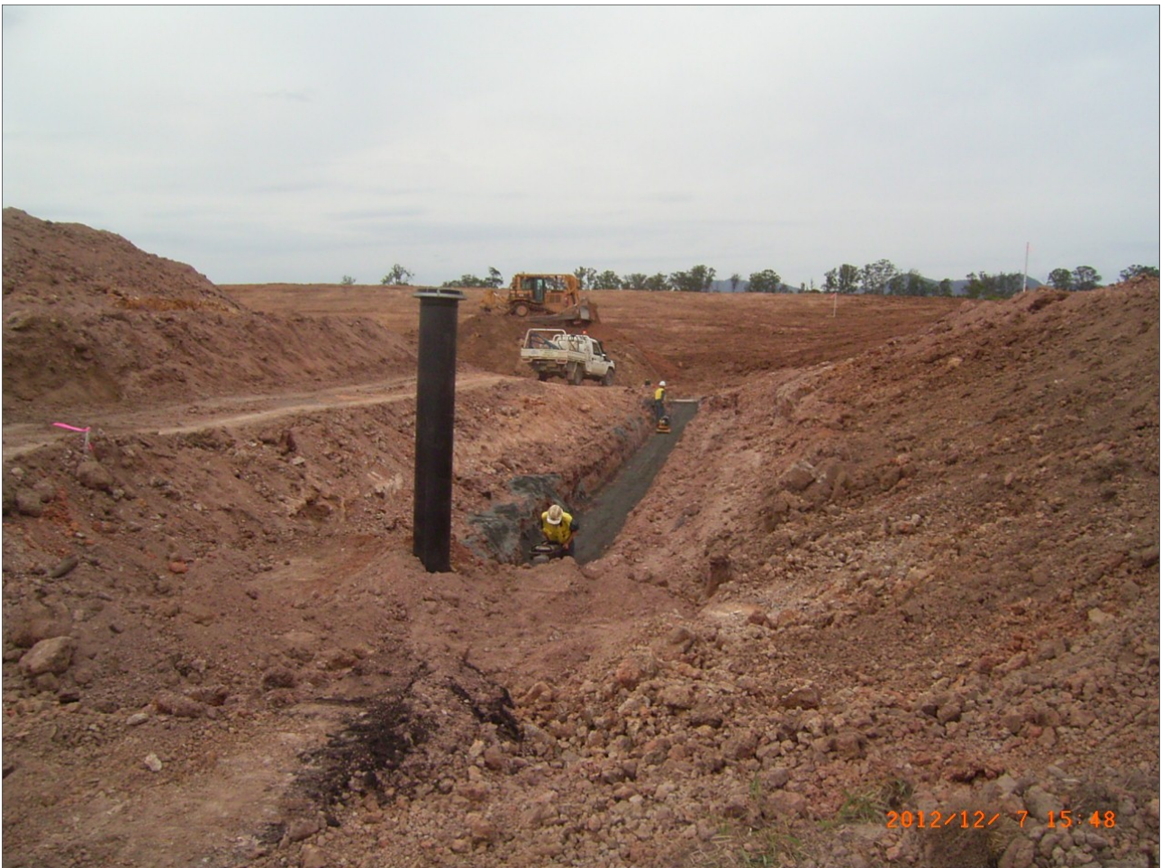
Horizontal pipe compaction done with a hand operated whacker packer until heavy compaction equipment could be used.
