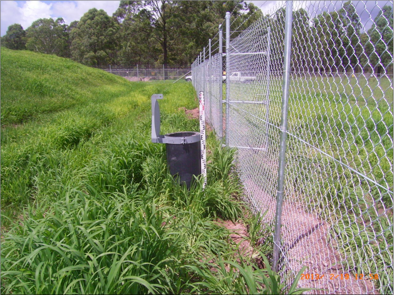
Position of leak detector to the dam wall and perimeter fence
