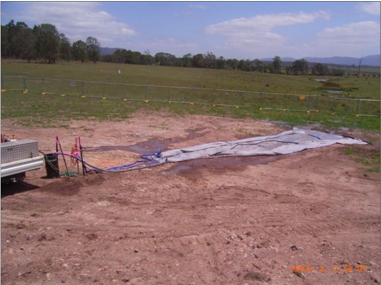
Pumping from the leak detector prior to the primary liner installation
