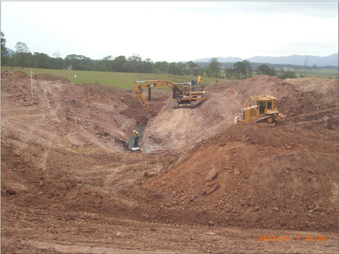
Leak detector installation using 5mm minus crusher dust with a 2% cement incorporation.
