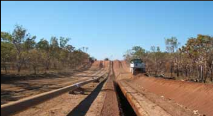
Photograph 3 Padding of pipe trench prior to lowering of pipe
