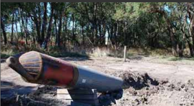
Photograph 7 Completed HDD operation with pipe having been pulled under river. (Note no damage to riparian vegetation in background)
