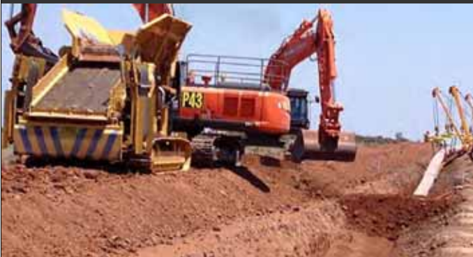
Photograph 5 Pipeline padding and trench backfilling. Lowering in of pipe in background
