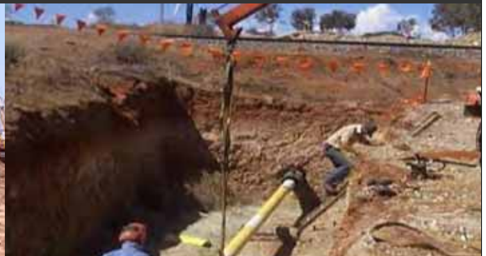
Photograph 6 Thrust boring
