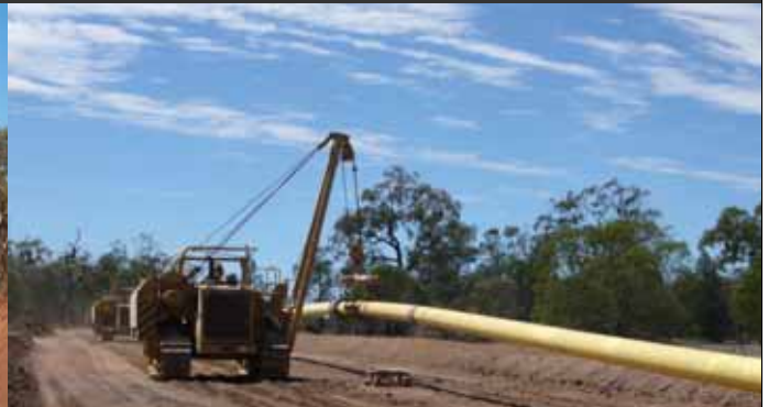
Photograph 4 Lowering of pipe
