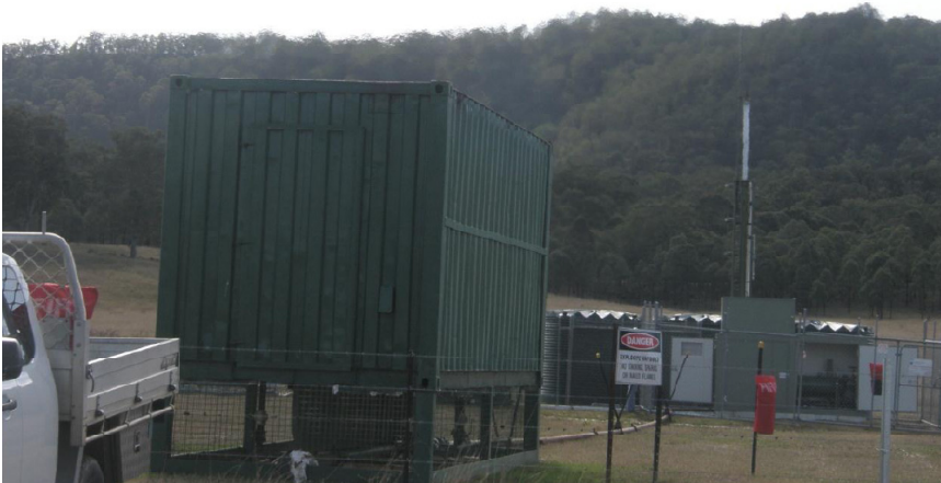
Photograph 2.2 AGL 20 ft flare facility – painted a colour to blend with the surrounding landscape
