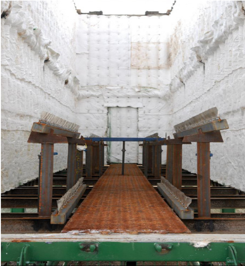
Photograph 2.3 AGL flare facility – internal view
