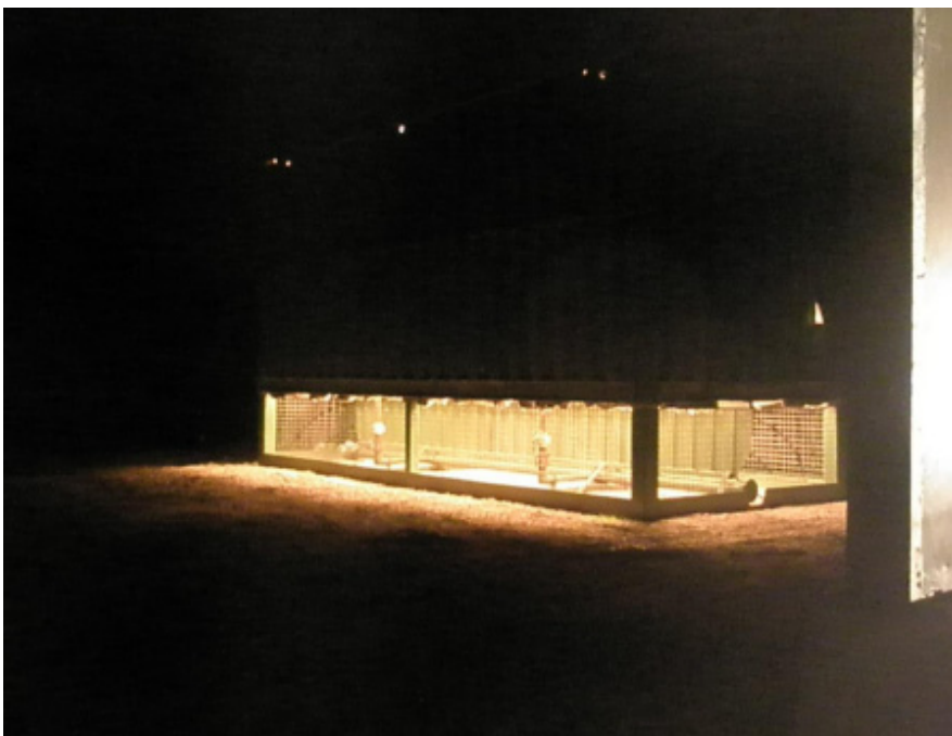
Photograph 2.4 AGL flare facility – operating at night with screening barrier in foreground on right
