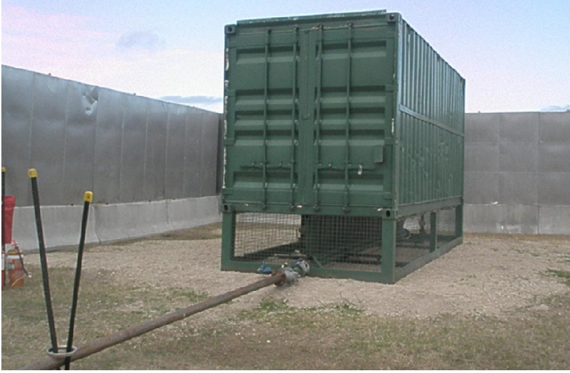
Photograph 2.1 AGL 20 ft flare facility – raised and enclosed around the flame
