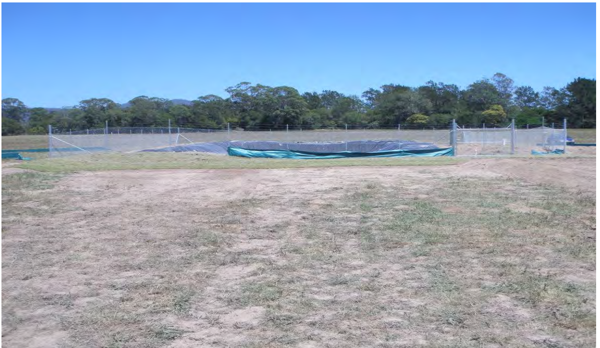
Plate 15. Catch Dam 2, diversion banks and temporary runoff & erosion protection
