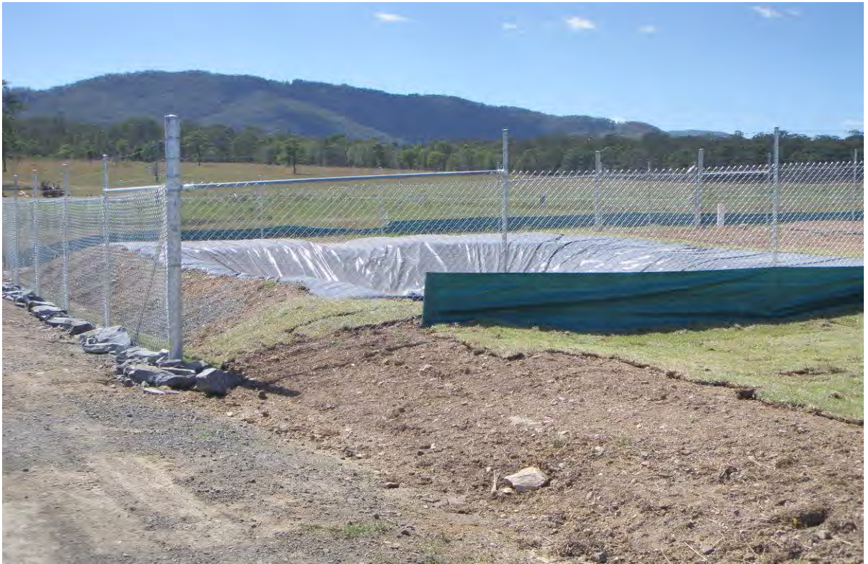
Plate 14. Catch Dam 1, diversion banks and temporary runoff & erosion protection
