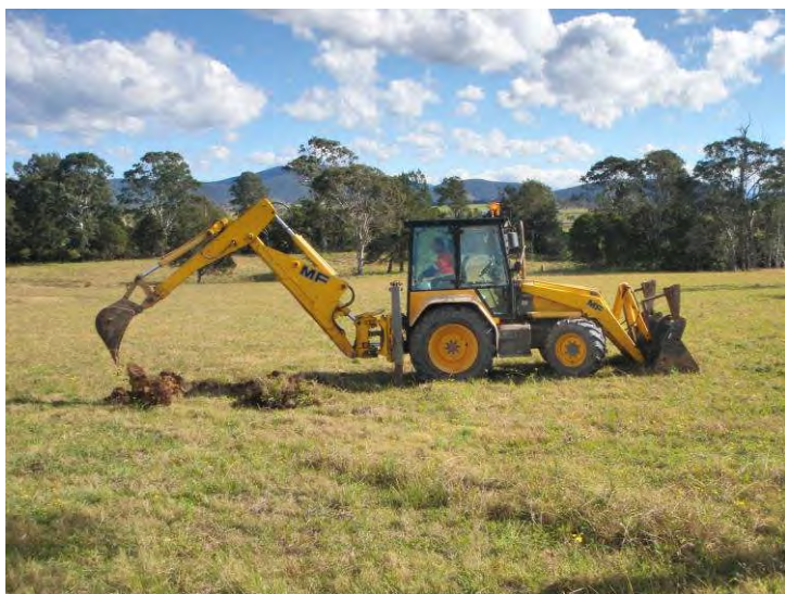
Plate 5. Digging test pits
