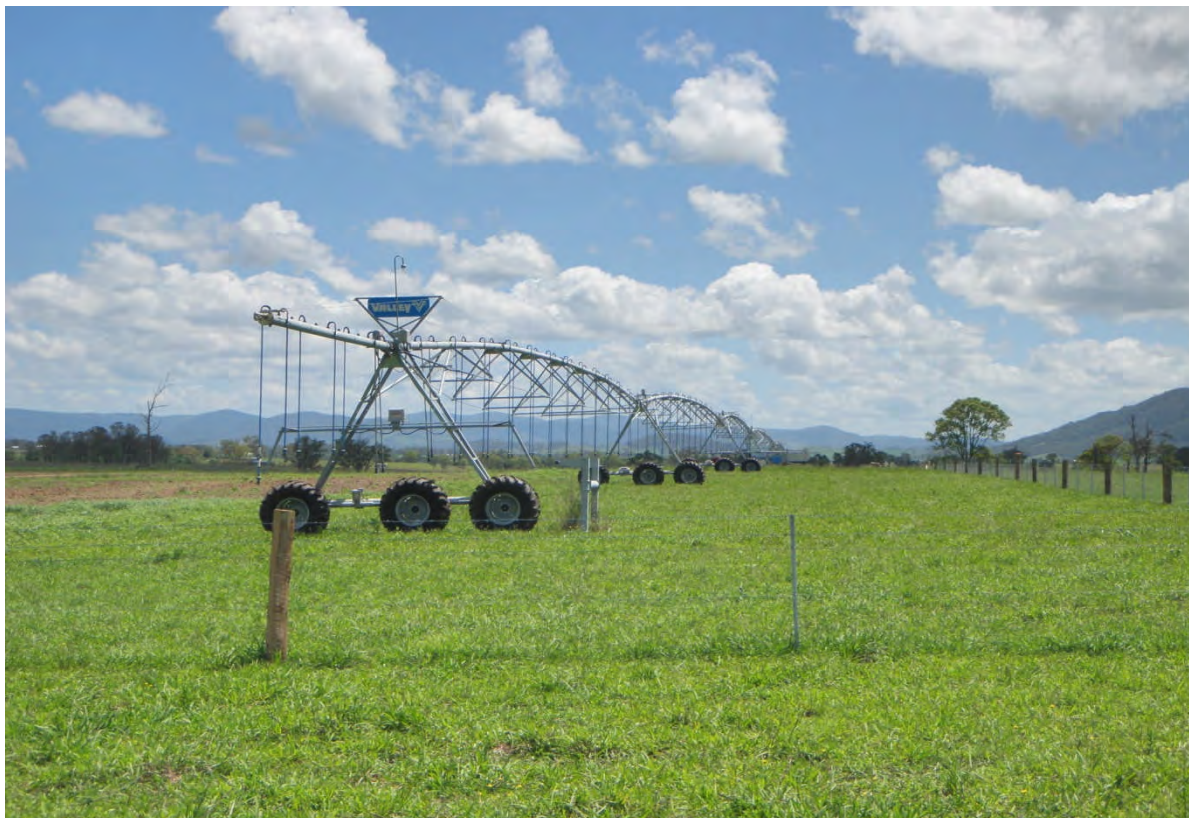
Plate 1. Low pressure overhead spray linear irrigator installed and ready for use on the Stage 1A irrigation area
