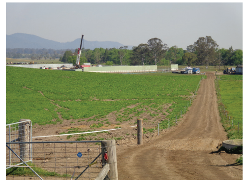
▲ Drilling at the Waukivory pilot well was recently completed.
