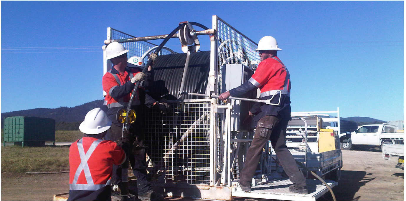
^Team purging deep monitoring bore
