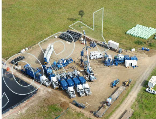
AGL fracturing operation in Gloucester
