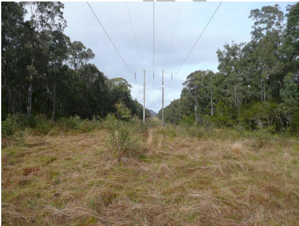
Plate 1: KP 66.8, which is typical of the existing environment at KP 59.8
