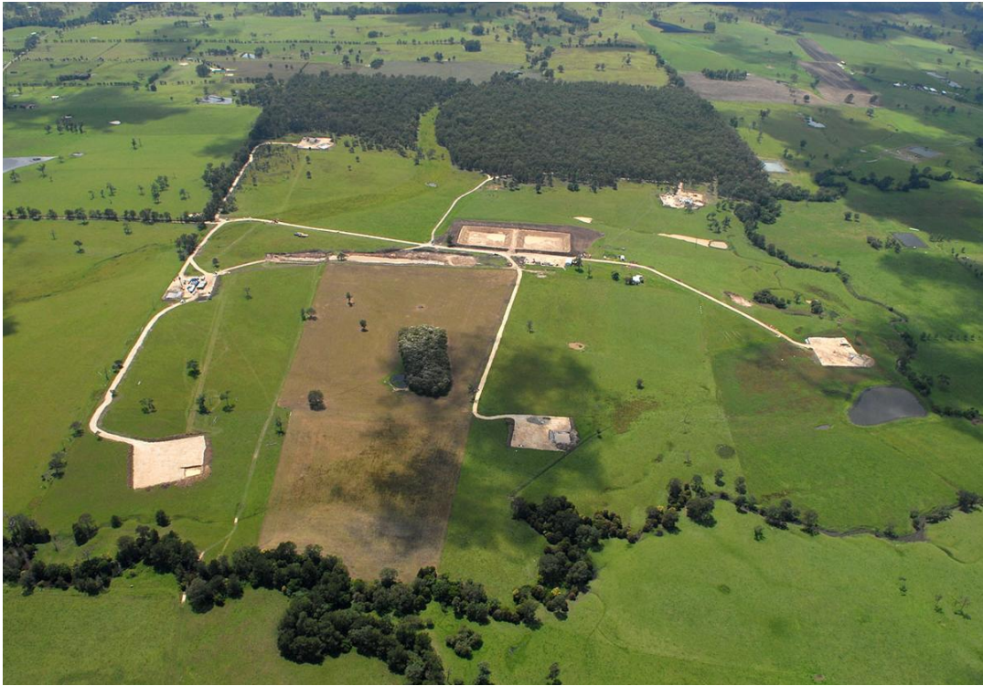
Figure 7: Well heads before initial rehabilitation on the Teidman property
