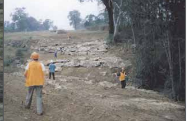
Photograph 6 Hand-broadcasting of seed along drainage line. Rock walls placed to assist with bank stability.
