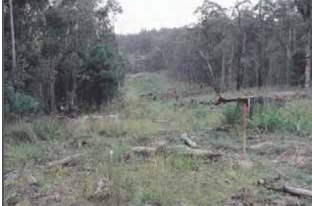
Photograph 4 Early establishment of revegetation through heavily vegetated area. Re-spreading of vegetation across easement evident.
