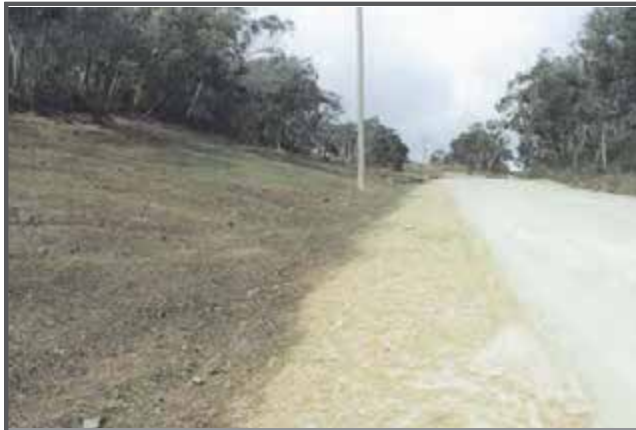
Photograph 1 Early regeneration of ground cover following hydro mulching along the roadside corridor.
