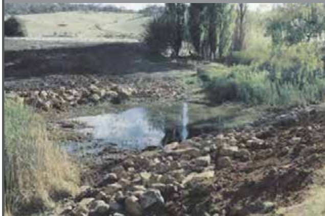
Photograph 7 Rehabilitation of open trenched creek crossing. Natural contours have been restored and rip rap placed to assist bank stability.
