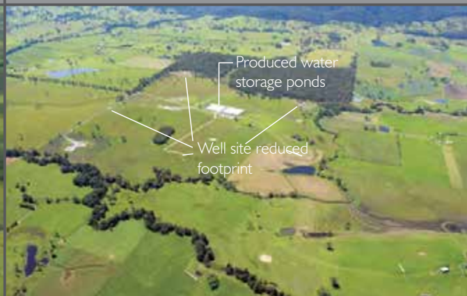
Photograph 11 Aerial photograph of the reduced and rehabilitated footprint (15x15m) for each well site at the Stratford Pilot
