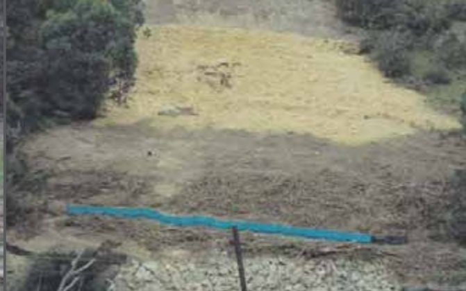
Photograph 5 Rehabilitation of an open trenched creek crossing. Hydro mulching rip rap and sediment and erosion control fencing present along creek line.
