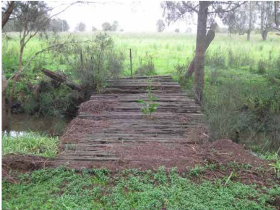
Plate P29: Bridge at LEH11
