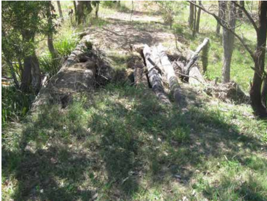
Plate P27: Bridge at LEH9
