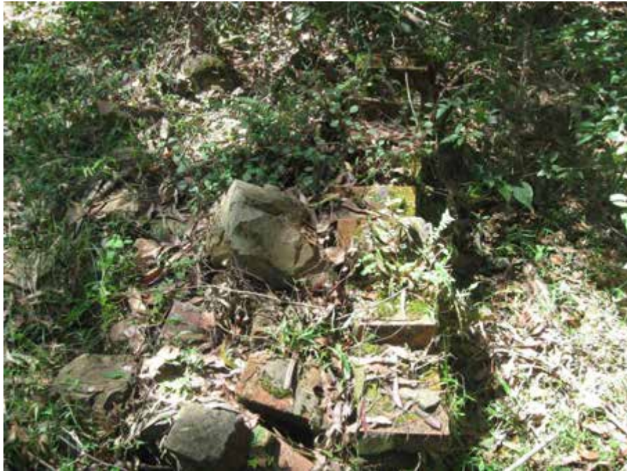
Plate P23: Pile of bricks at LEH5
