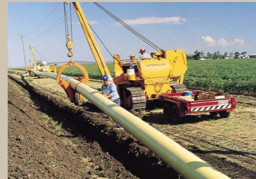
Laying pipeline
