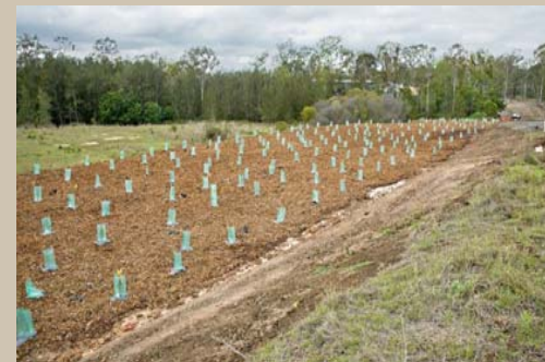
Pipeline easement during restoration
