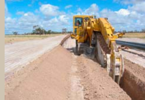
Trenching during Pipeline Construction
