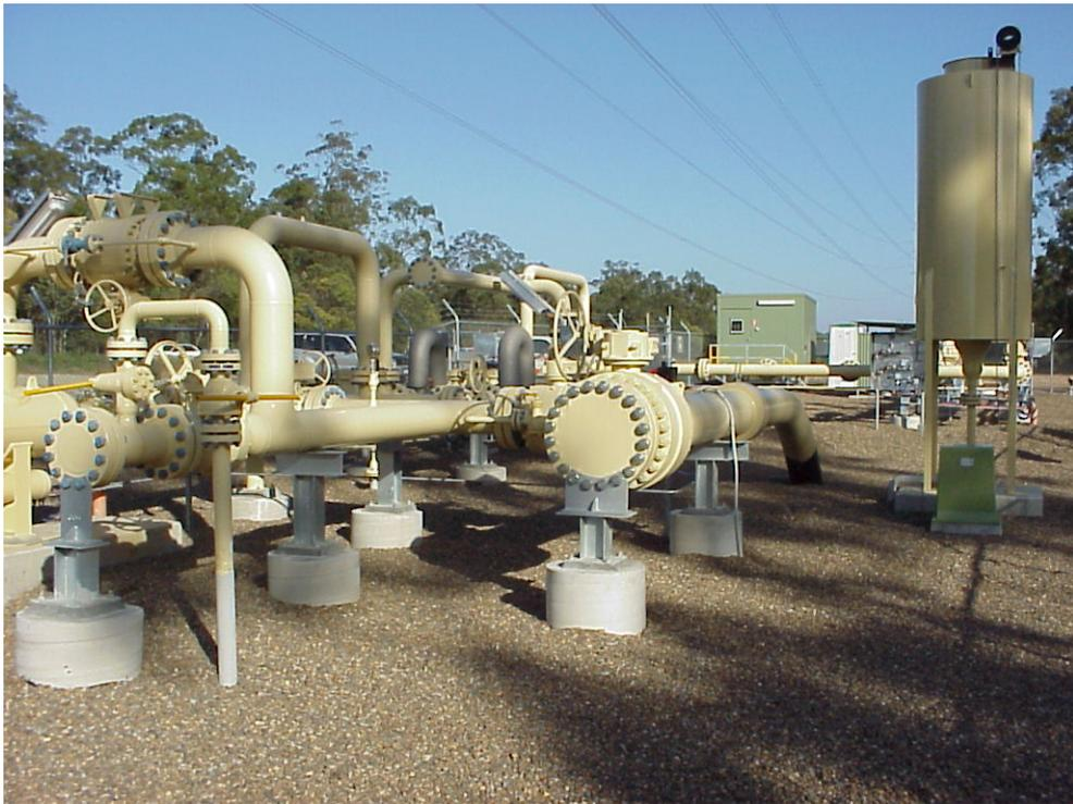
**Plate 1** – Valve station, typical internal arrangement
