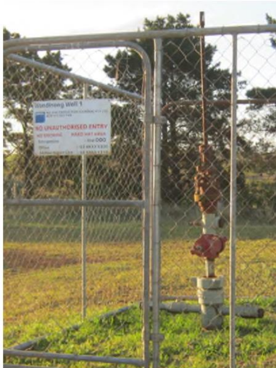
WG01 Prior to Cut and Cap
