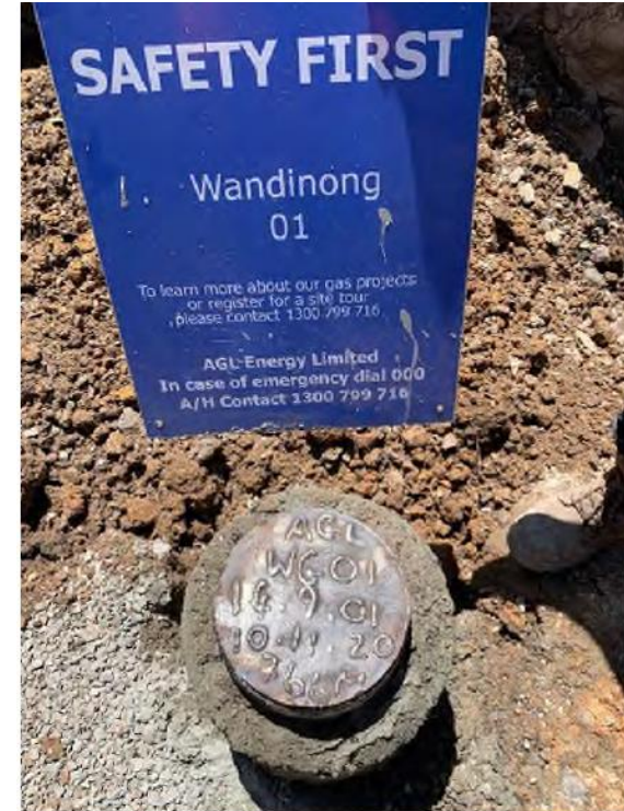
WG01 Well Head P&A Plate installed
