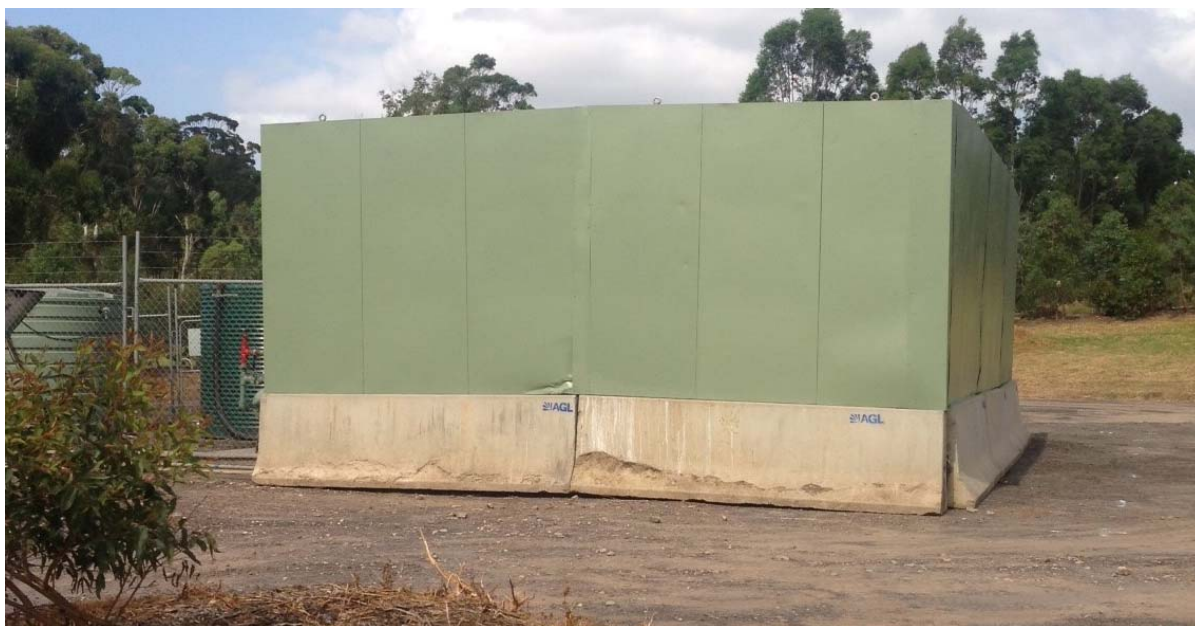
Figure 5 Noise Walls at SF20
