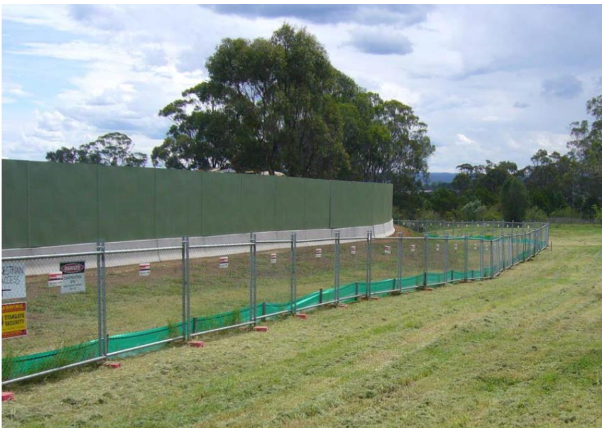
Figure 5.1 Noise wall used during construction activities at previous sites
