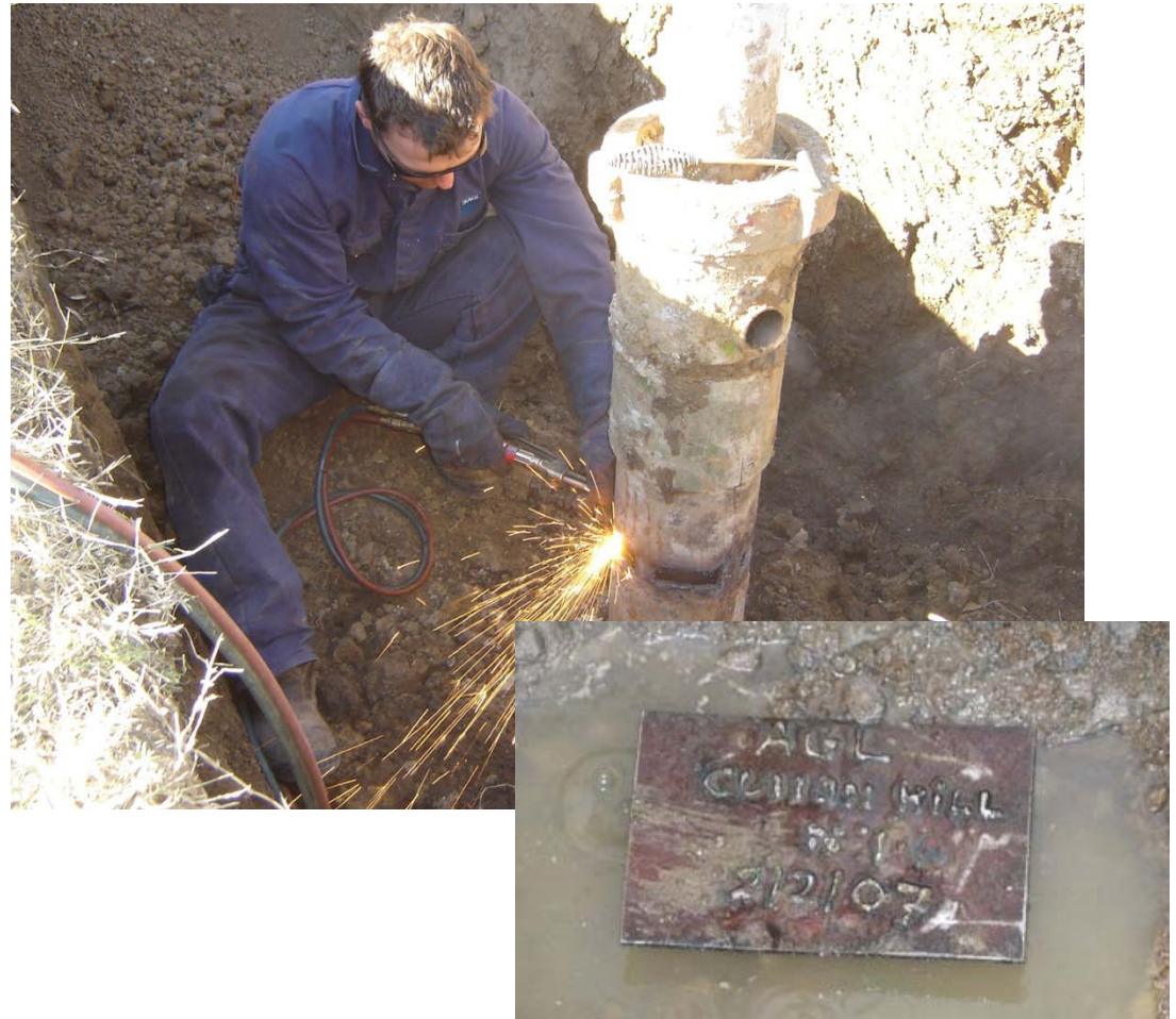
An exploration core hole during plug and abandonment (above)
