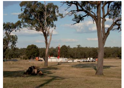
▲ Drilling rig used for a core hole.
